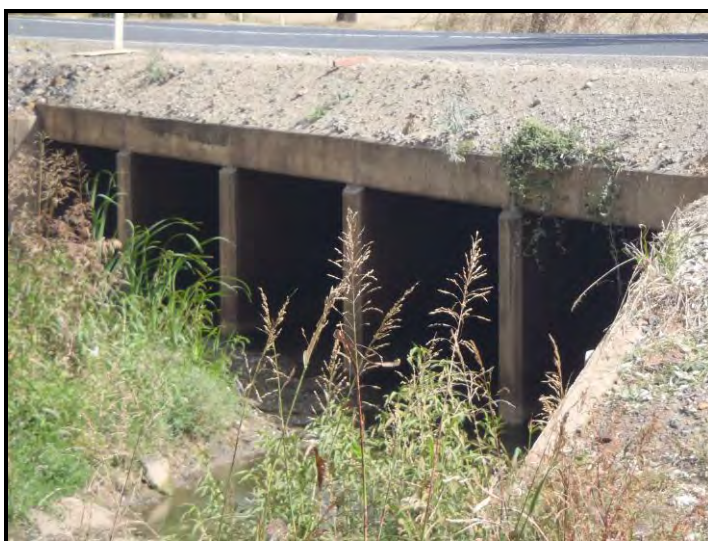
Figure 7: Gregory Highway crossing flow structure
