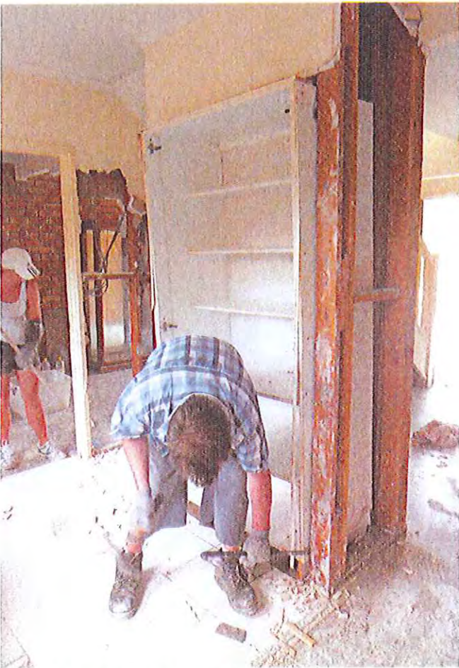
removing kitchen pantry
