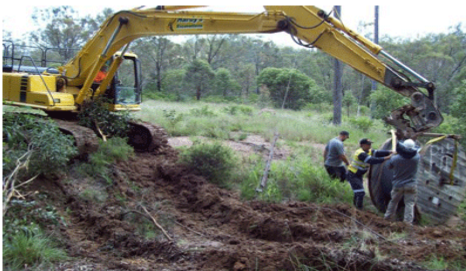
Picture: Engineers repairing inter-city cable at Helidon, QLD 2011
