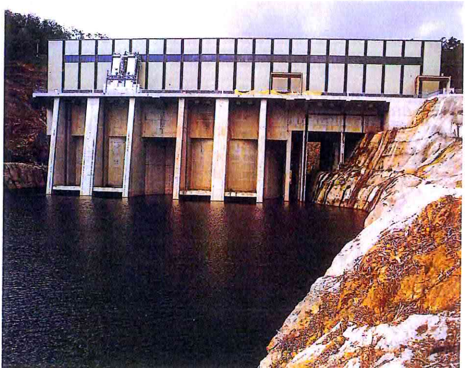
The power station viewed from the bank of the tail bay off Wivenhoe Dam.
