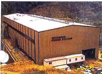
Assembly bay building almost completed late in 1983.
