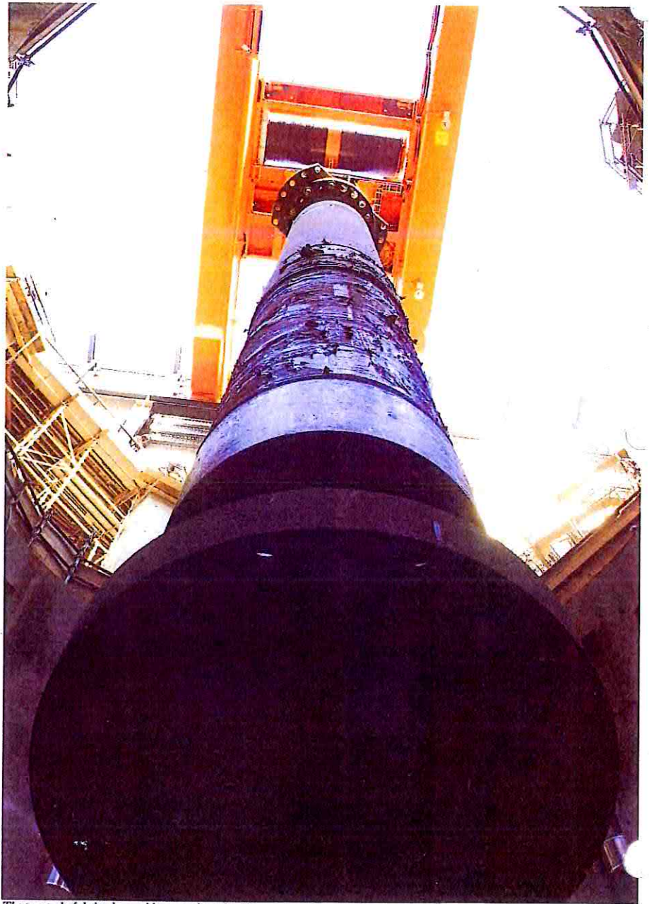
The pump shaft being lowered by crane into the silo.
