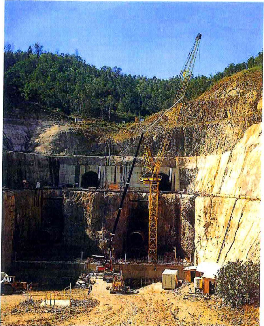
Early construction mid-1980 showing foundations and installation of pump branch pipes.
