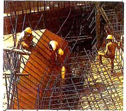
Construction work was accelerated to achieve completion by mid-1984.
