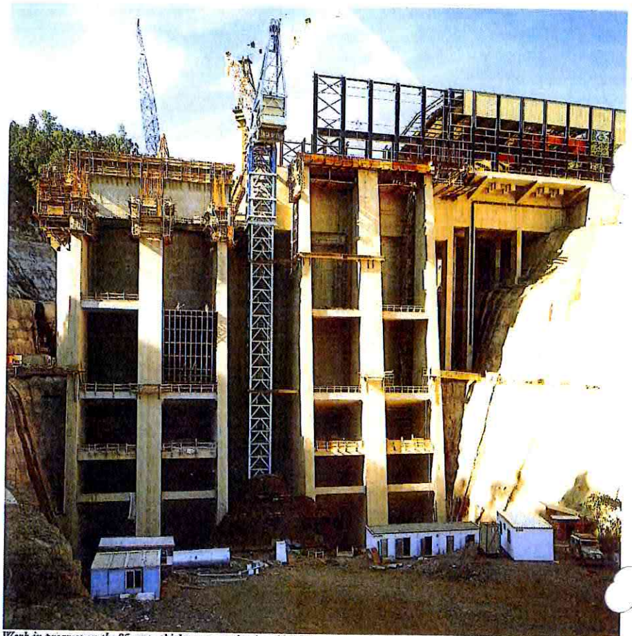
Work in progress on the 95-metre-high power station in mid-1982.
