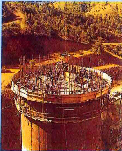
Construction of a Split-Yard Creek Dam intake tower.
