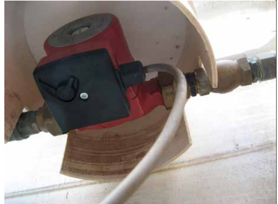
Close up of hot water recirculation pump that needed to be replaced
