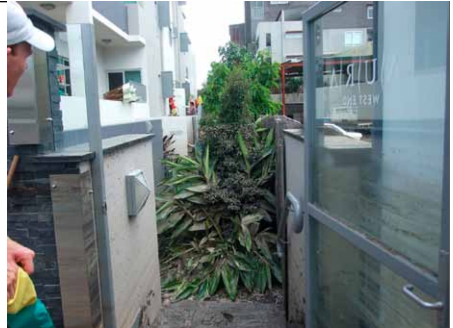
Street entrance down some steps at the side of the building leading to the fire stairs halfway along and showing the water heater room (white walls) in the middle
