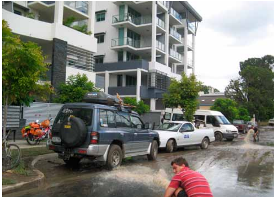
Cleaning the mud outside Aura Apartments on 14/01/11 at 12.04 pm
