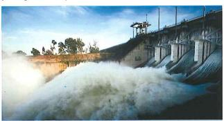
As soon as Wivenhoe Dam's flood storage compartment begins to fill, it has to be carefully emptied in order to make room for additional heavy rainfall events that may occur. Wivenhoe Dam's flood storage compartment can fill in less than three days following heavy rainfall. This highlights the need for strategic management of dam levels. Controlled releases consider the following flood factors: catchment runoff below the dam wall, urban runoff and river levels.
