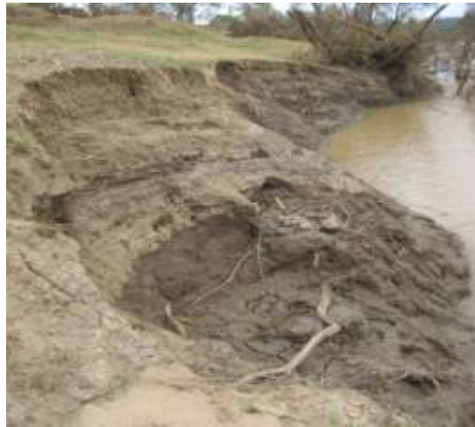
Photo 002 – Jan 11 Fence & Tree Destruction
