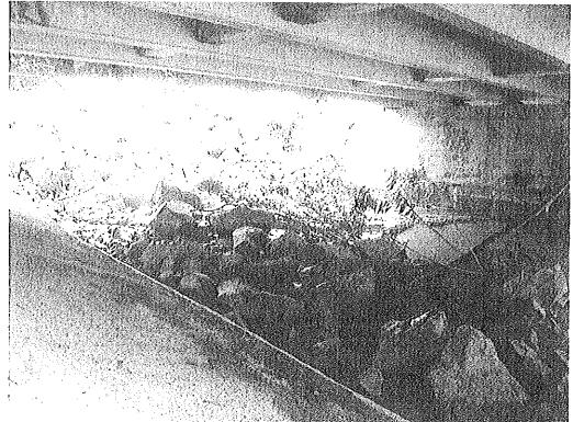
Figure 8: Under the A. J. Wylie Bridges at Abutment A looking upstream it is seen that flow through span 1 of the north bound structure is blocked by the upstream channel geometry,
