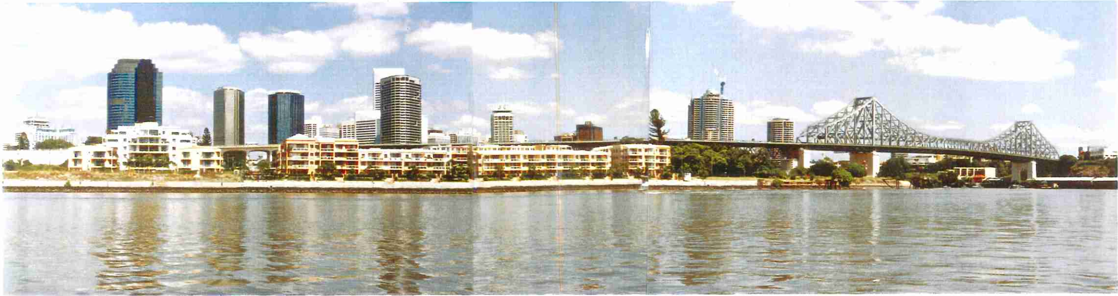
STRUCTURE 7-STORY BRIDGE (LOOKING UPSTREAM)
