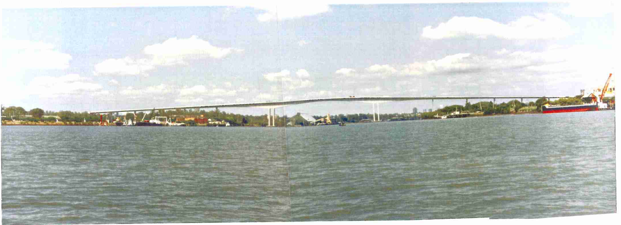
STRUCTURE 8-GATEWAY BRIDGE (LOOKING UPSTREAM)
