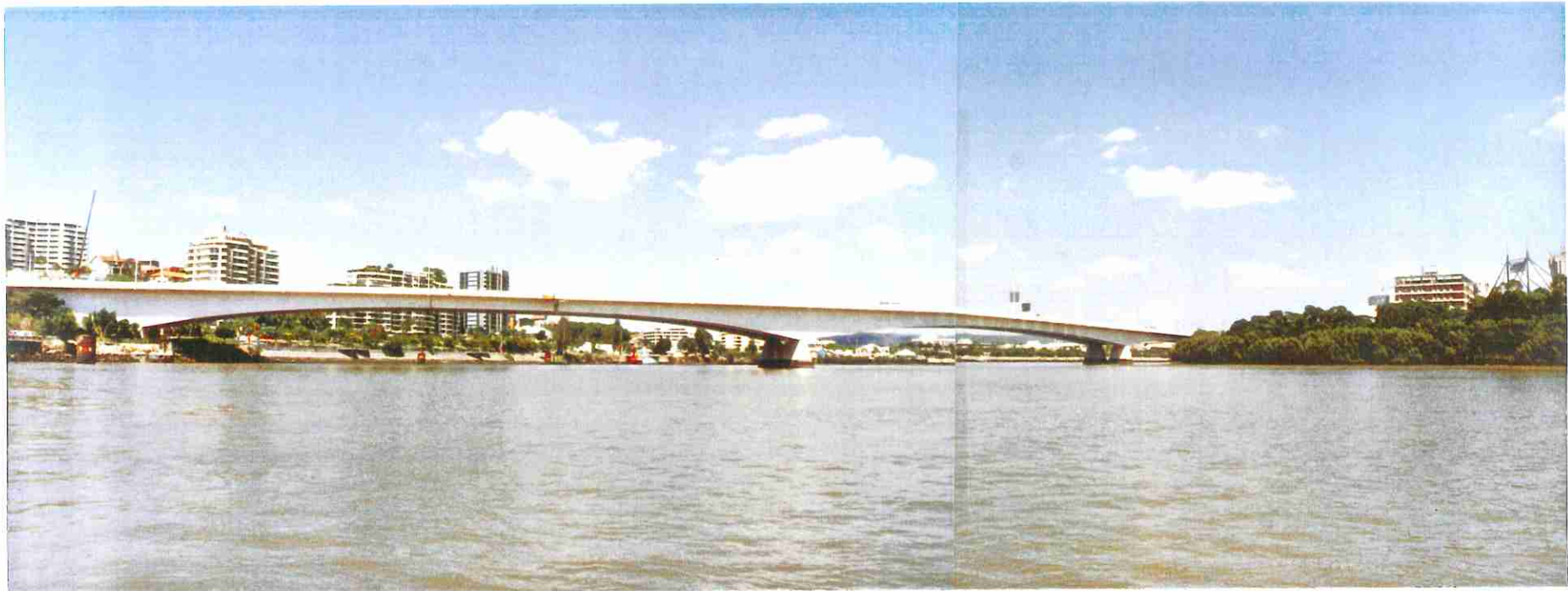
STRUCTURE 6-CAPTAIN COOK BRIDGE (LOOKING UPSTREAM)
