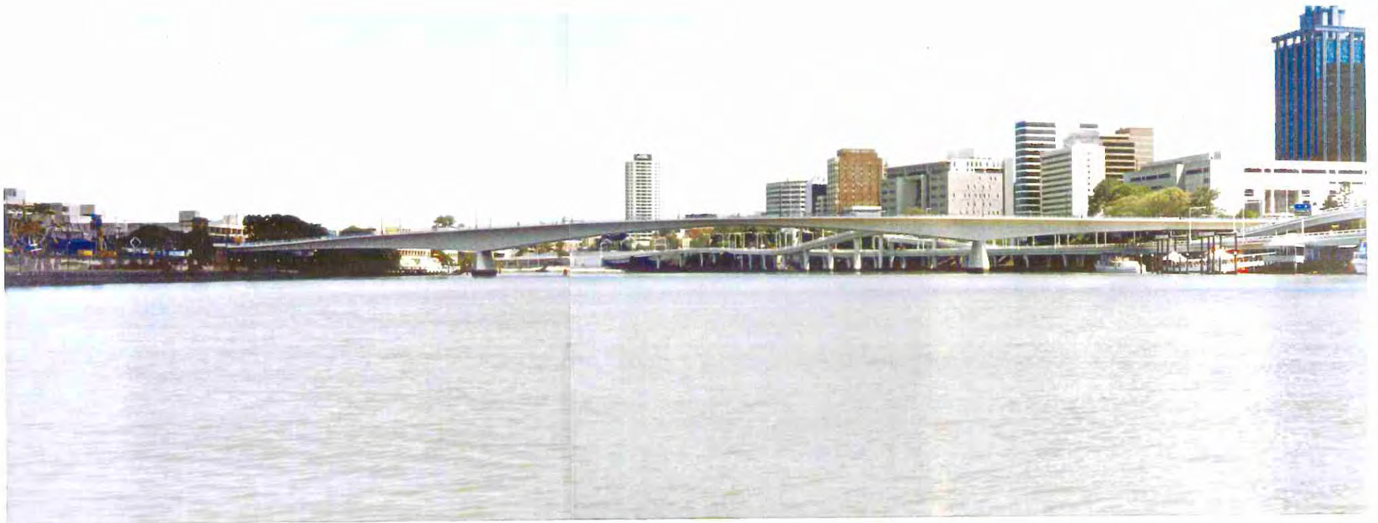
STRUCTURE 5-VICTORIA BRIDGE (LOOKING UPSTREAM)
