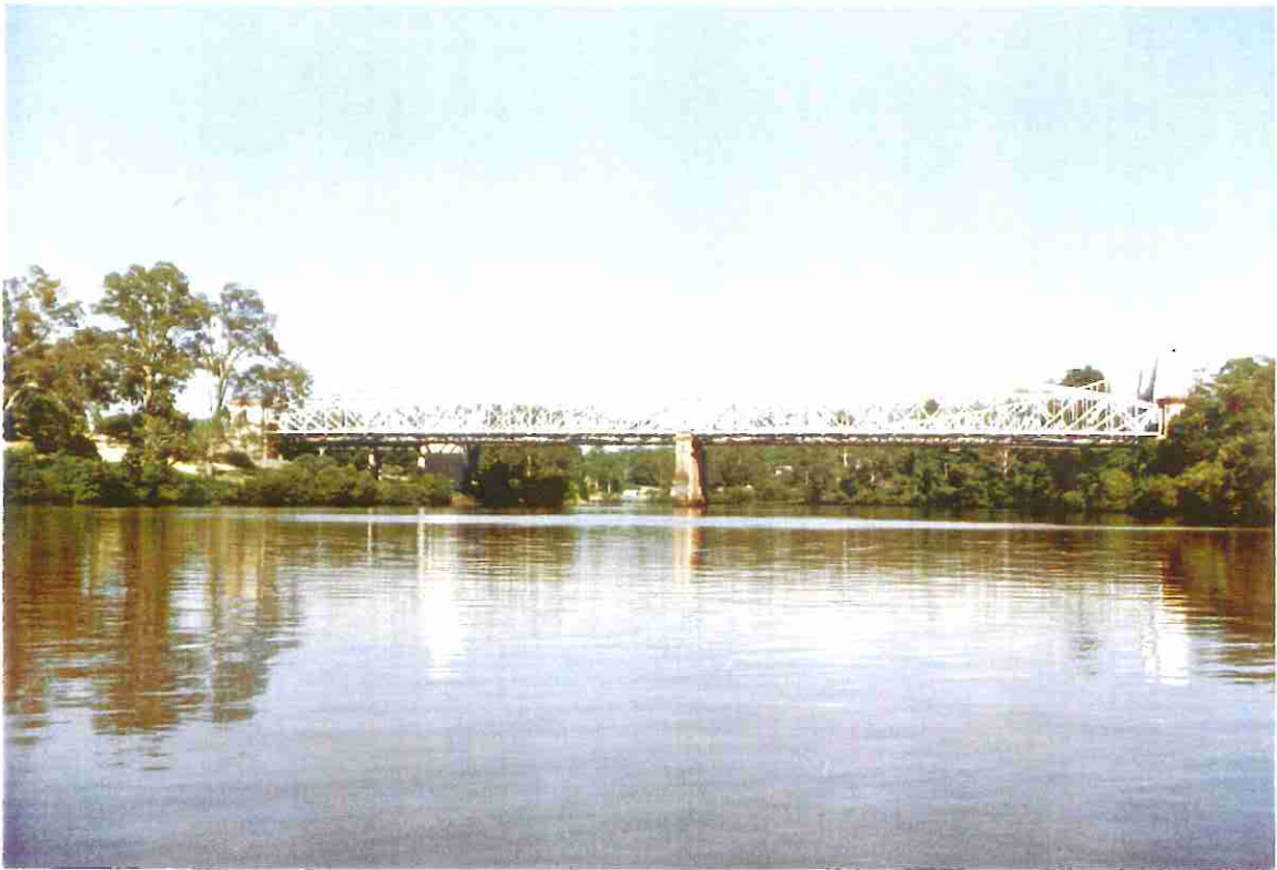
STRUCTURE 2-INDOOROPILLY BRIDGES (LOOKING UPSTREAM)
