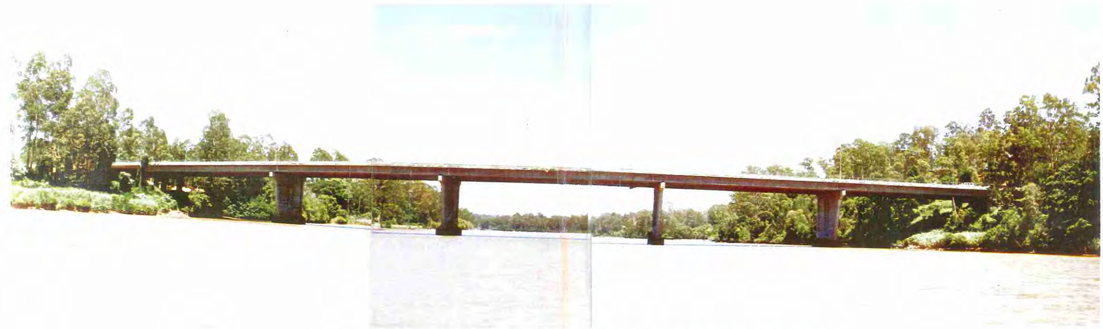
STRUCTURE 1-CENTENARY BRIDGE (LOOKING UPSTREAM)
