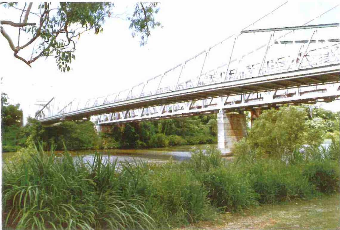
STRUCTURE 2-INDOOROPILLY BRIDGES (LOOKING DOWNSTREAM)
