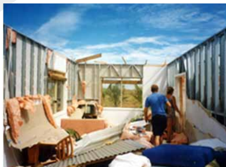
Picture 4 – inadequate roof truss anchorage
