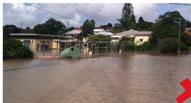
Photo 1: Example of an older, non-resilient substation design
