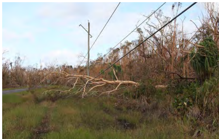
Photo of powerlines damaged by fallen vegetation in Tully Heads, courtesy of Ergon Energy
