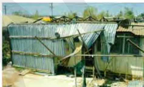
Picture 3 – inadequate batten to rafter connections (common in older housing)
