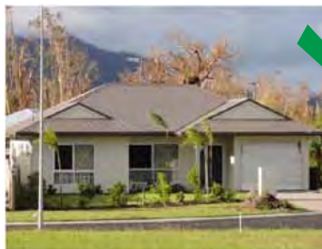
Picture 1 – roof has resisted loads near the design wind load in spite of minor debris damage and roller door failure
