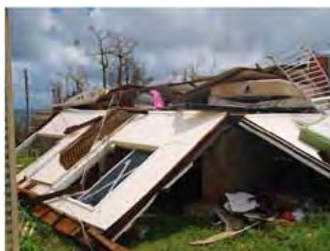
Picture 5 – inadequate tie down through the entire structure
