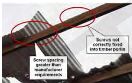
Picture 2 – roofing fasteners not installed in accordance with manufacturer's recommendations
