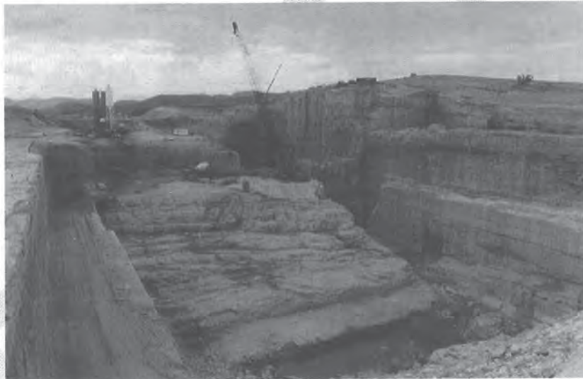
Photo 7- Wivenhoe Outlet and Spillway Plunge Pool Construction
