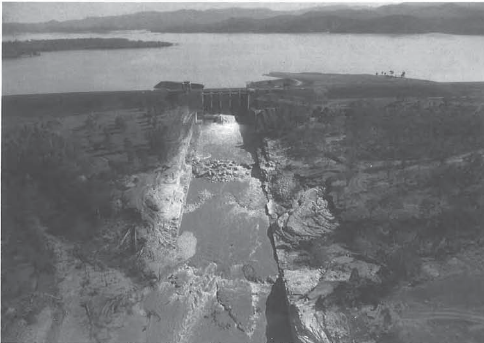
Photo 2- Wivenhoe Outlet Channel and Spillway Post January 2011 Flood
