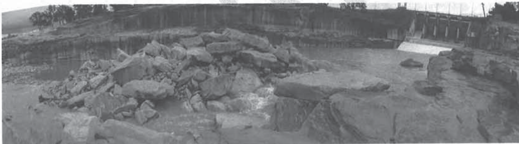
Photo 5- Wivenhoe Outlet Channel and Spillway Post January 2011 Flood
