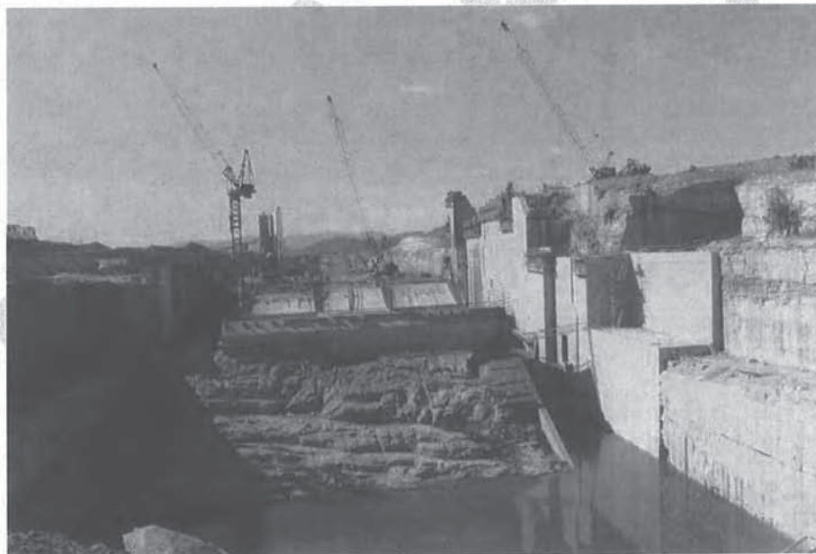
Photo 11- Wivenhoe Outlet and Spillway Plunge Pool Construction
