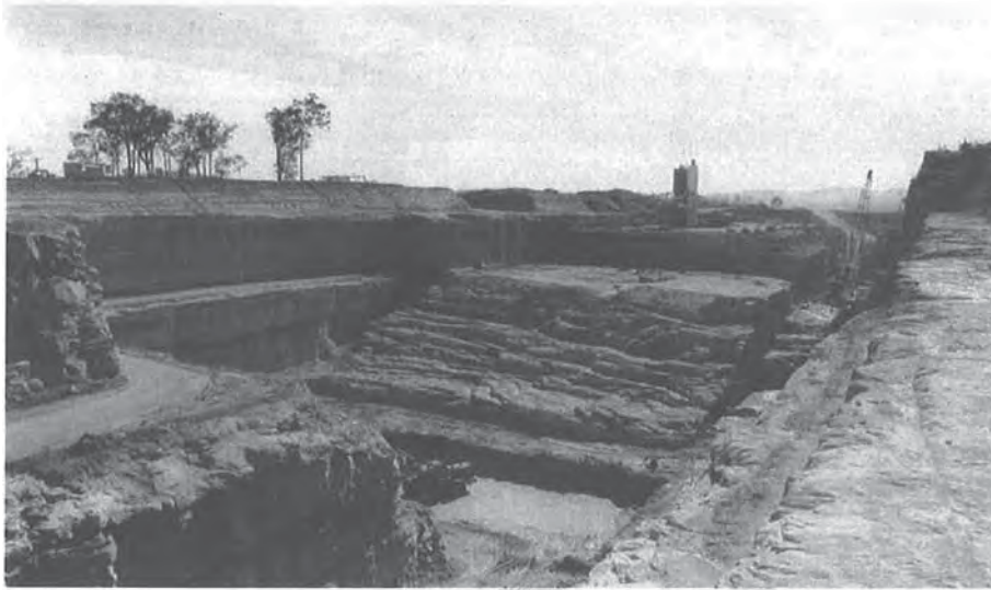
Photo 8- Wivenhoe Outlet and Spillway Plunge Pool Construction
