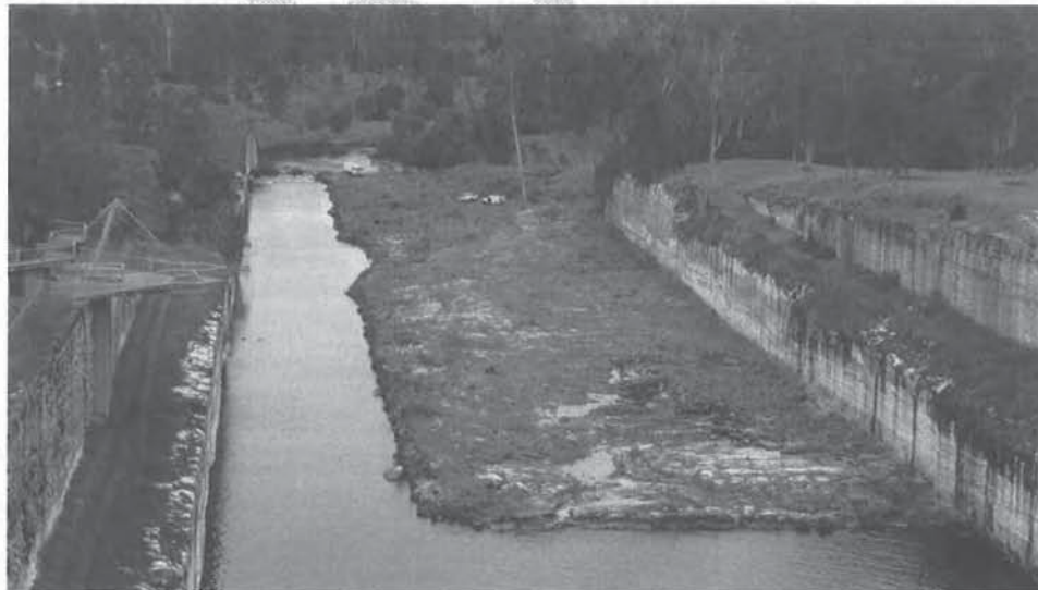
Photo 3- Wivenhoe Outlet Channel and Spillway Prior to January 2011 Flood
