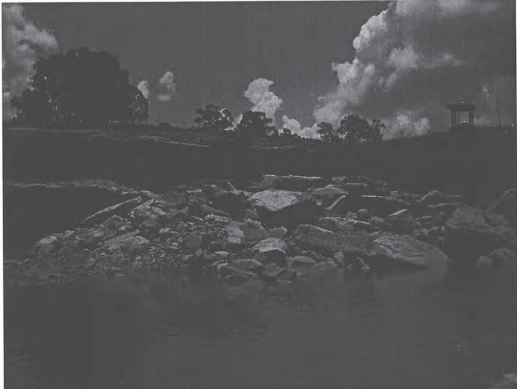
Figure 3 Sandstone Block Bank from downstream
