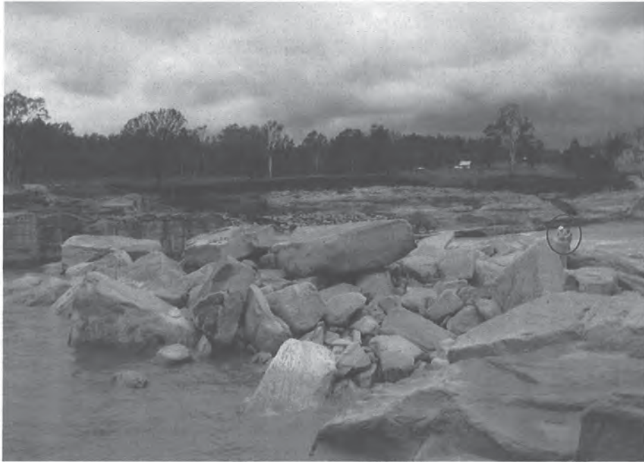
Photo 6- Wivenhoe Outlet Channel and Spillway Post January 2011 Flood
