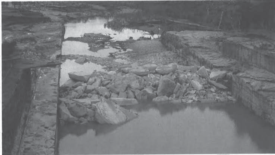
Photo 4- Wivenhoe Outlet Channel and Spillway Post January 2011 Flood
