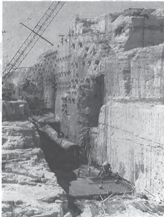
Photo 9- Wivenhoe Outlet and Spillway Plunge Pool Construction
