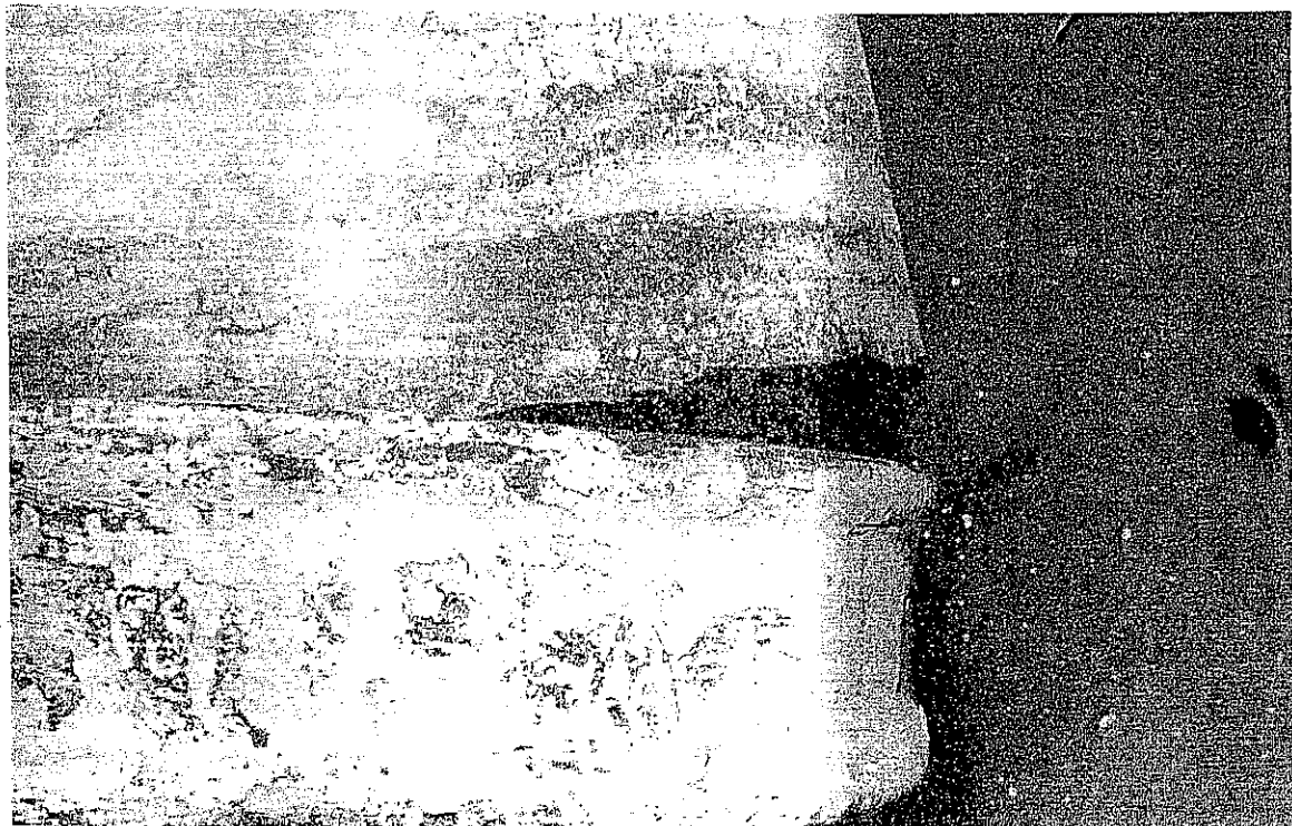
36" dia. Lock Bar water main across Moggill Creek showing pipe end pulled out of lead jointed collar. 234.
