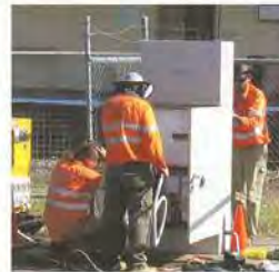
Employees work to repair Goodna station after flooding
