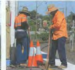
Workers re-lay CCTV cables at Goodna station
