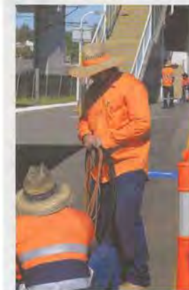
Workers relay cable at Goodna station.
