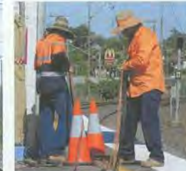
Workers rebuy CCTV cables at Goodna station
