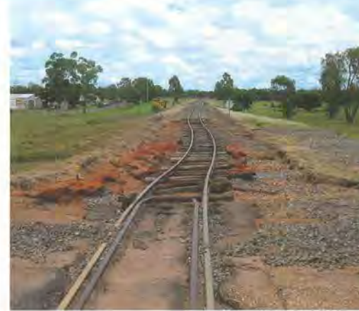
Damaged track between Barcaldine and Alpha on the south-west line
