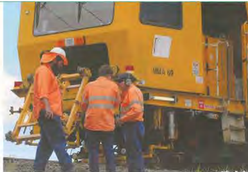
Workers assist with the tamping of ballast on track near Rowwood.
