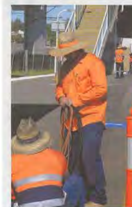
Workers relay cable at Goodna station.
