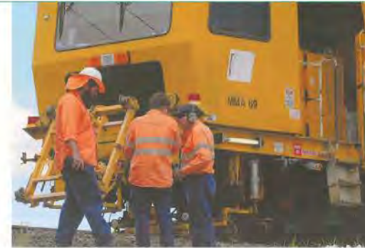
Workers assist with the tamping of ballast on track near Rowwood.
