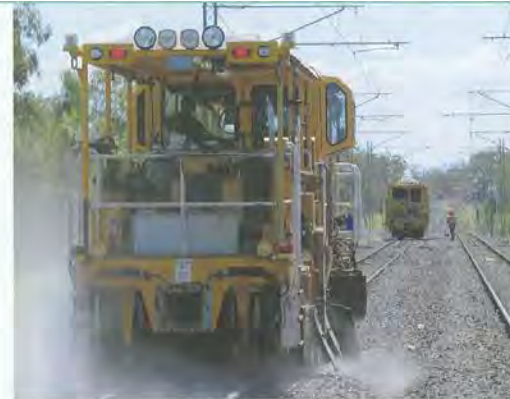
A ballast regulator re-profiles ballast on the line near Rosewood
