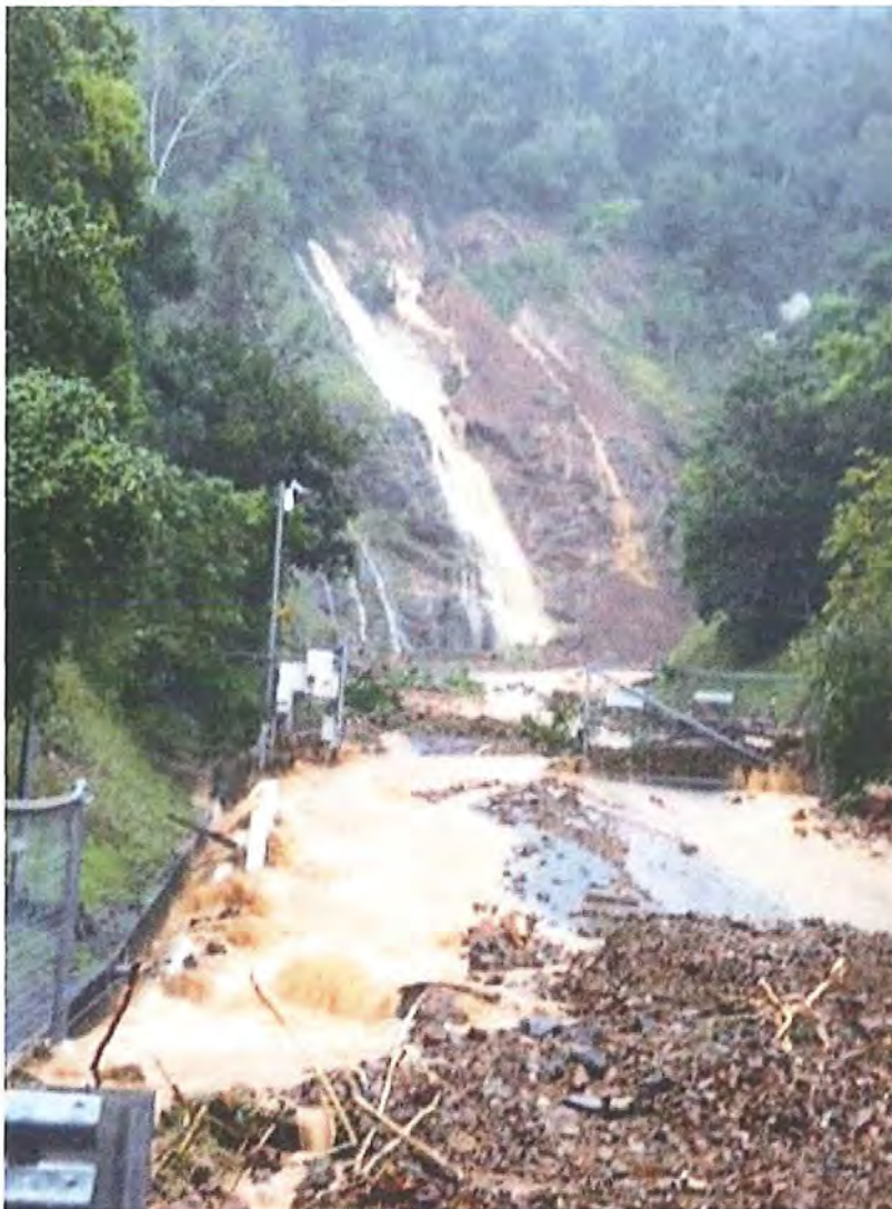
WPS - Main Access Road – 11 January 2011
