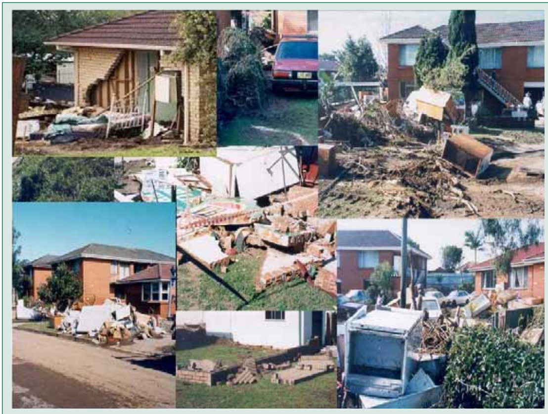
Figure 30b Flooding can cause catastrophic damage
