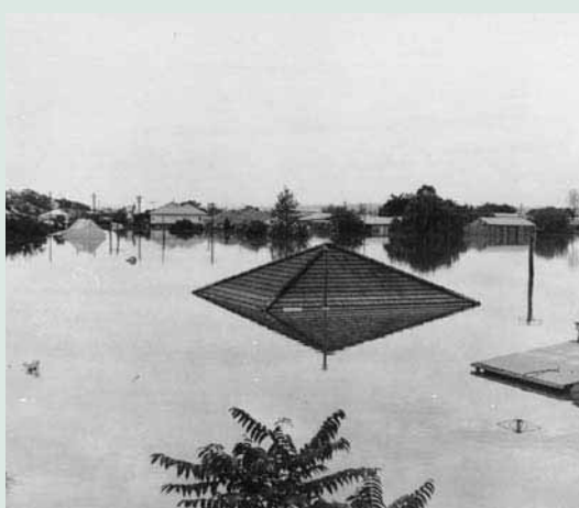
Figure 14 A house in Windsor inundated above the eaves
