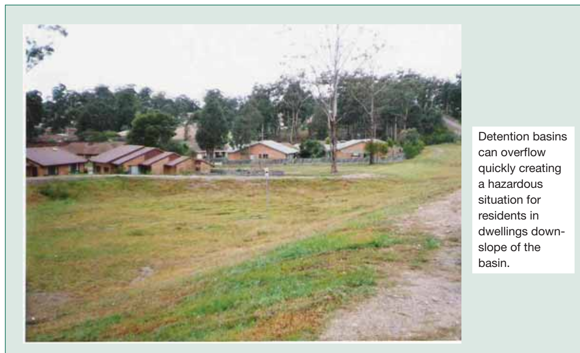
Figure 62 Detention basin upstream of dwelling houses
