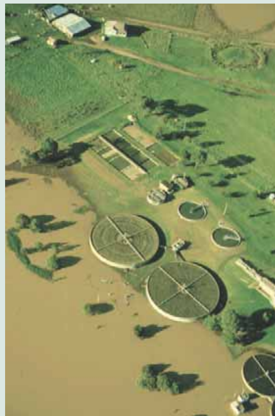
Figure 58 Sewage Treatment Plant on the floodplain
