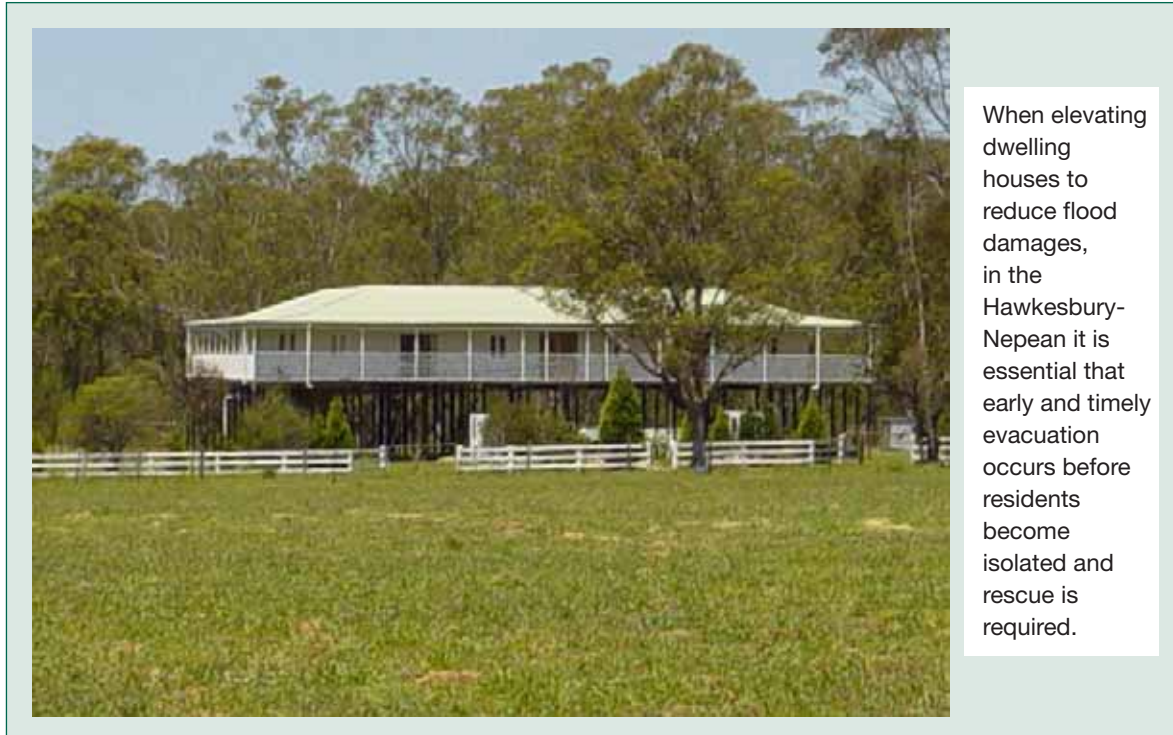
Figure 65 Elevated house on flood prone land
