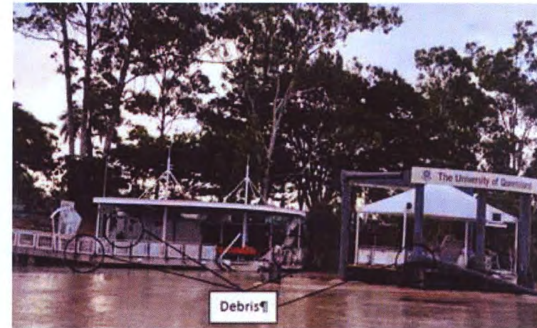
Figure 88: Failed Sydney Street Ferry Terminal
