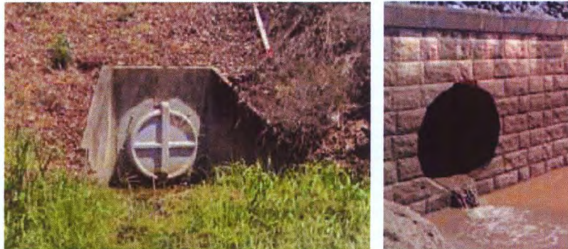
Figure 35: Outlet Pipe Non-return Device
