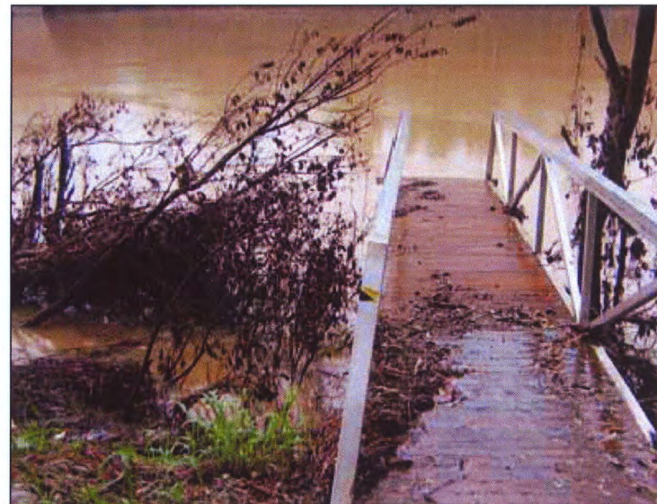
Figure 91: PT2008 – Part of Gangway, pontoon and piles washed away
