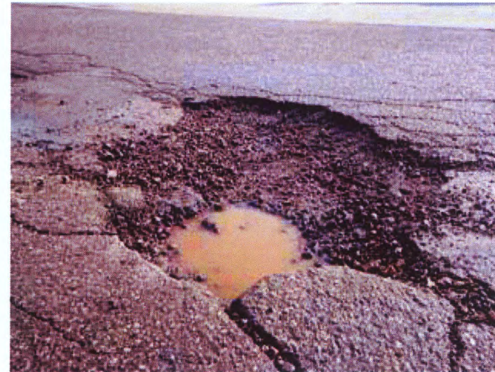
Figure 18: Pavement cracking leading to a pothole
