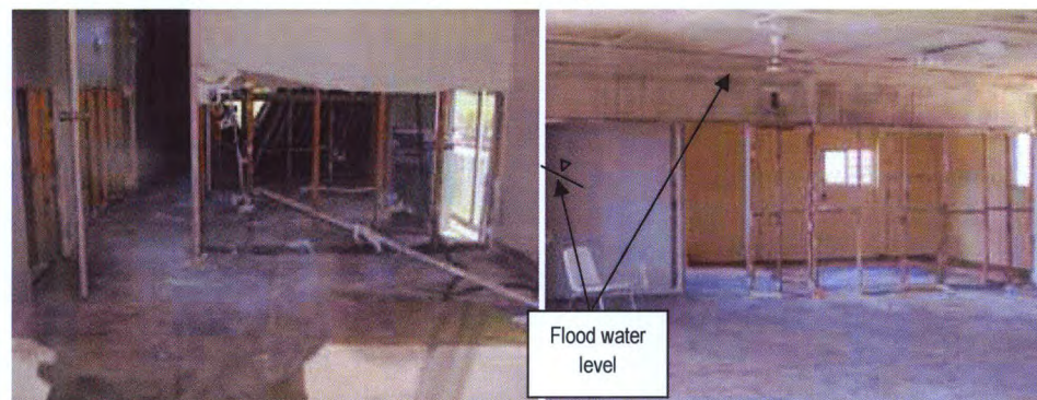
Partially inundated flood damage to internal cladding and frame Fully inundated flood damage to internal cladding and frame
