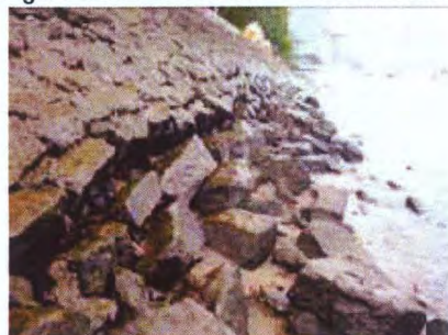
Figure 52: Prior Condition of Flood Damaged Riverwalls
