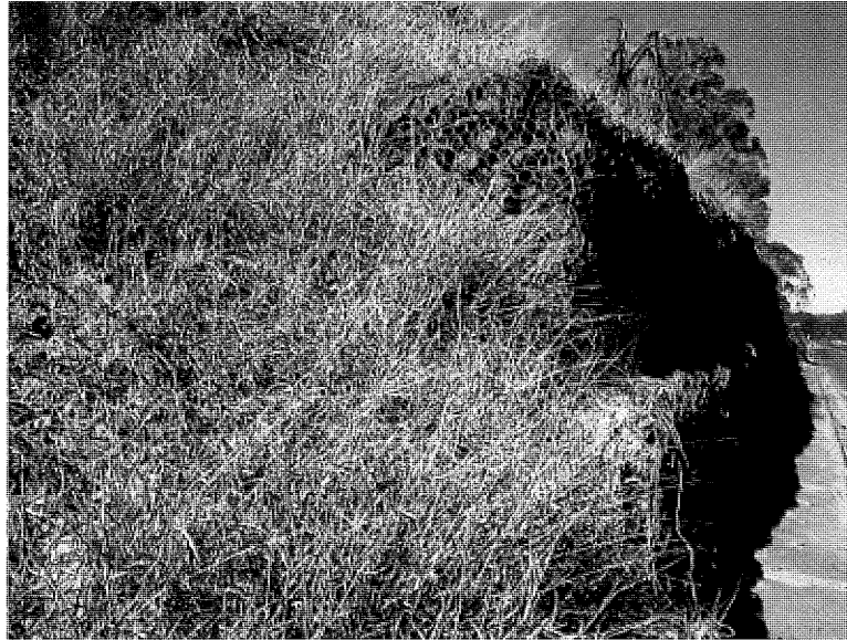
Figure 22: Example of gabions used to stabilise road cutting near Fernvale, Brisbane Valley.
