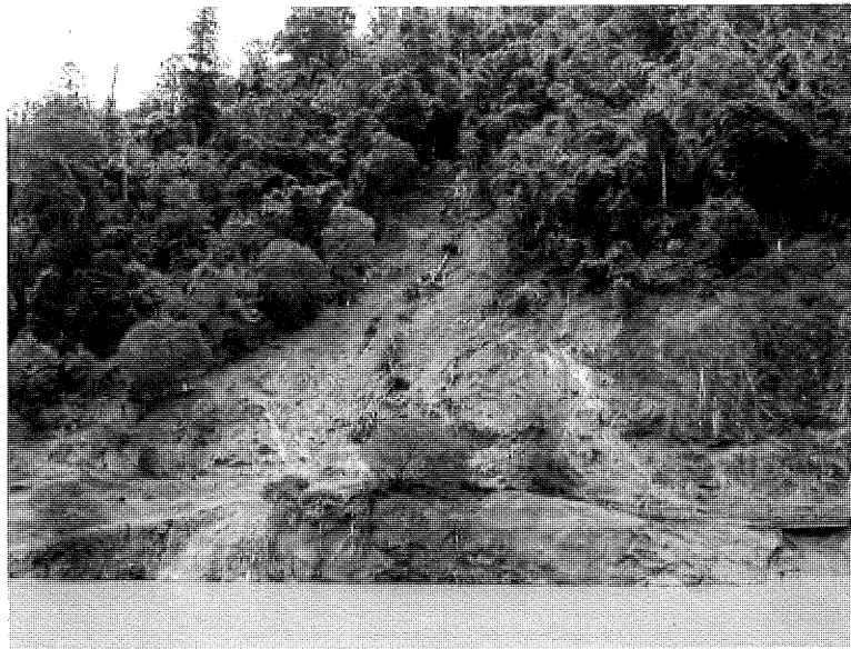
Figure 11: Slip located to the north of the pump intake area.
