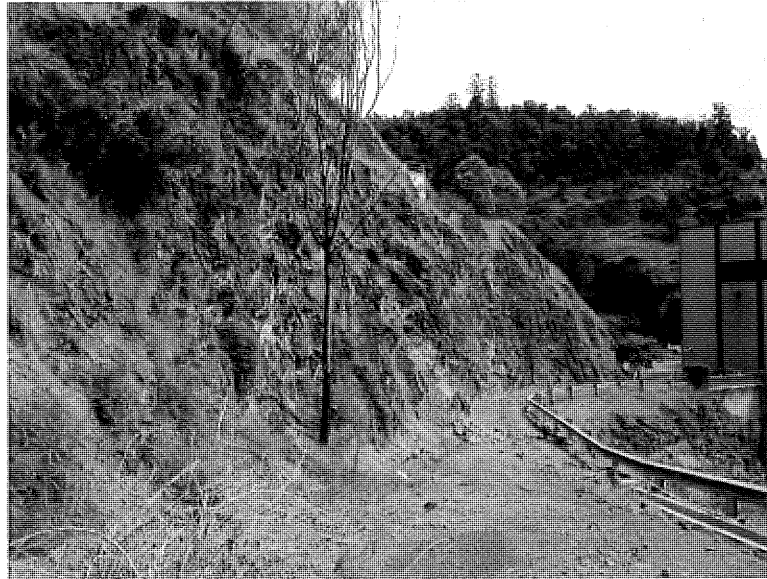
Figure 7: Over slip in soil in access track area.
