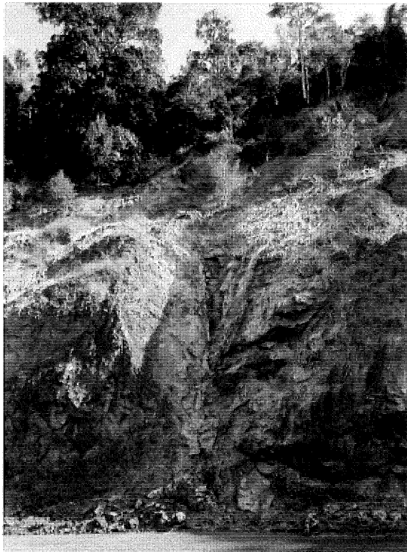
Figure 20: Preferred discharge zone, eroding weak rock along intersecting joints.
