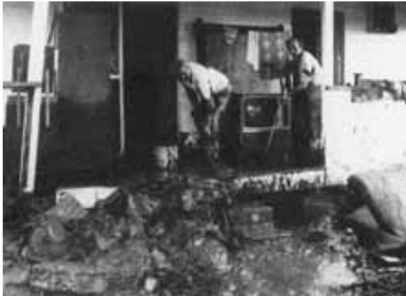
PLATE 5 – Lismore 1974 (Clean up of debris)
