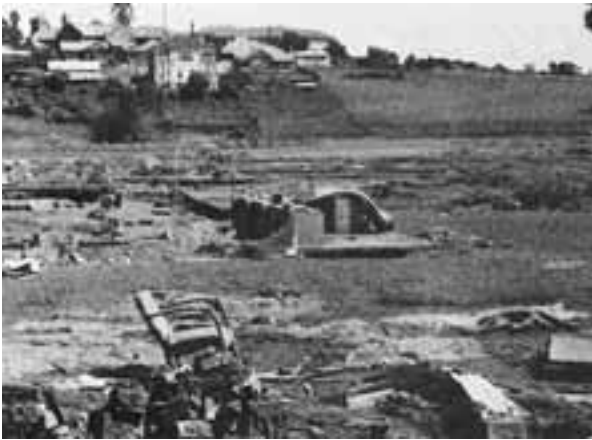
PLATE 3 - Mount Pleasant Street, Maitland, 1955 (20 houses stood in this street before the flood)
