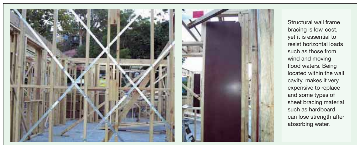
Figure 85 Durable frame bracing
