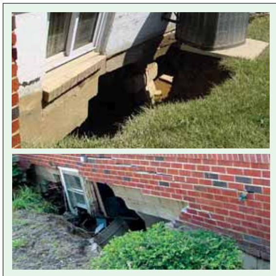
Figure 16 Collapse of walls due to hydrostatic pressure
