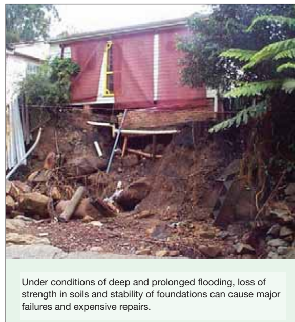
Figure 42 Undercutting from erosion
