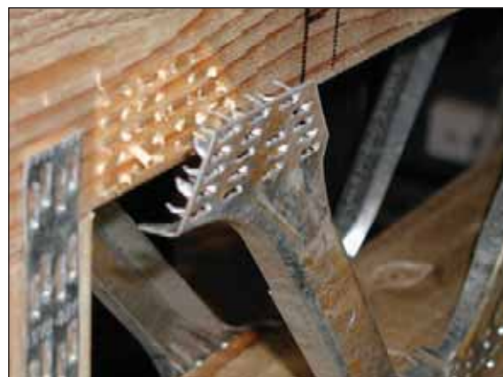
Figure 77 Beam failure
