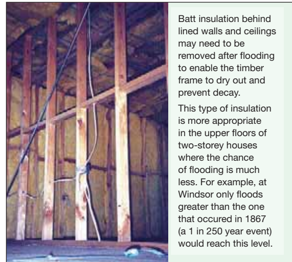
Figure 96 Problems with batt insulation
