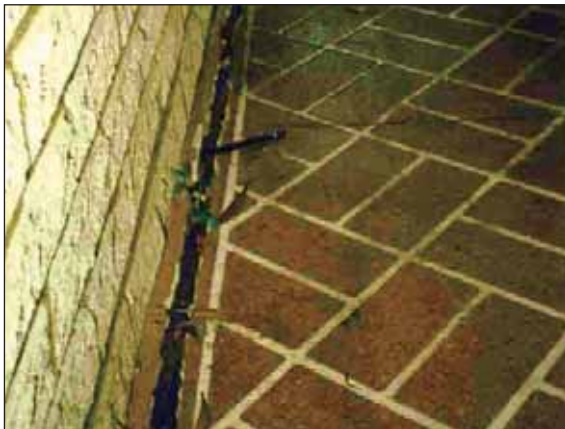
Figure 120 Brick wall bowed inwards due to water force
