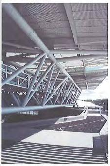
The existing concealed clip roof requires through-fastening to ensure it can withstand high winds.
