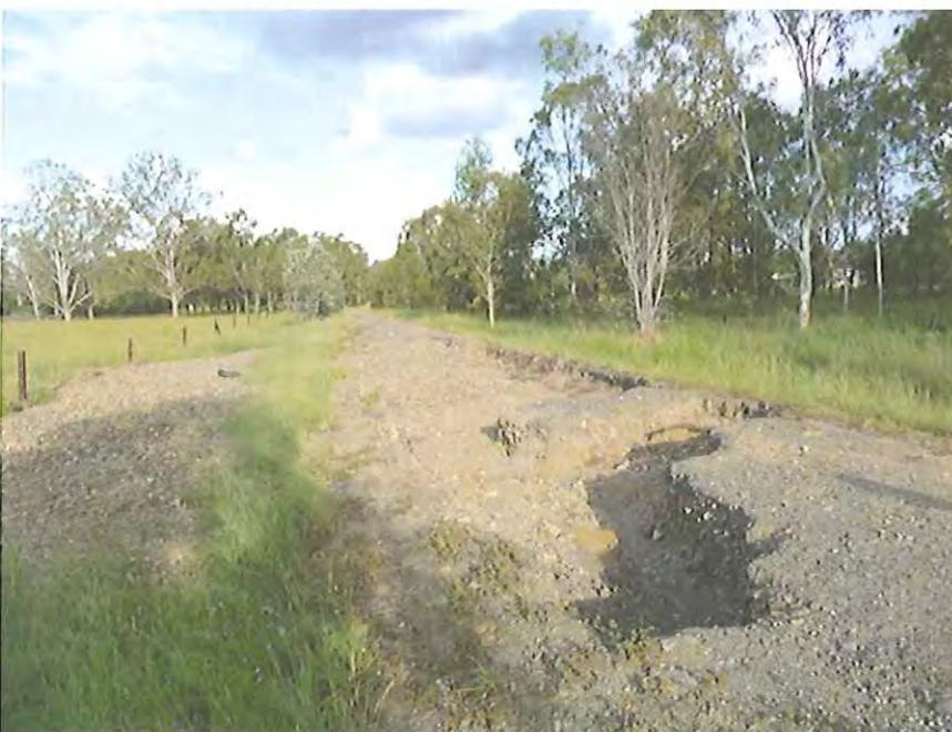
**Photograph A10** – Another example of severe erosion of the Old Brisbane Valley Rail Line (further to the west).
