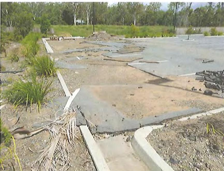
**Photograph A4** – Looking upstream across damaged car park pavement towards the damaged detention basin
