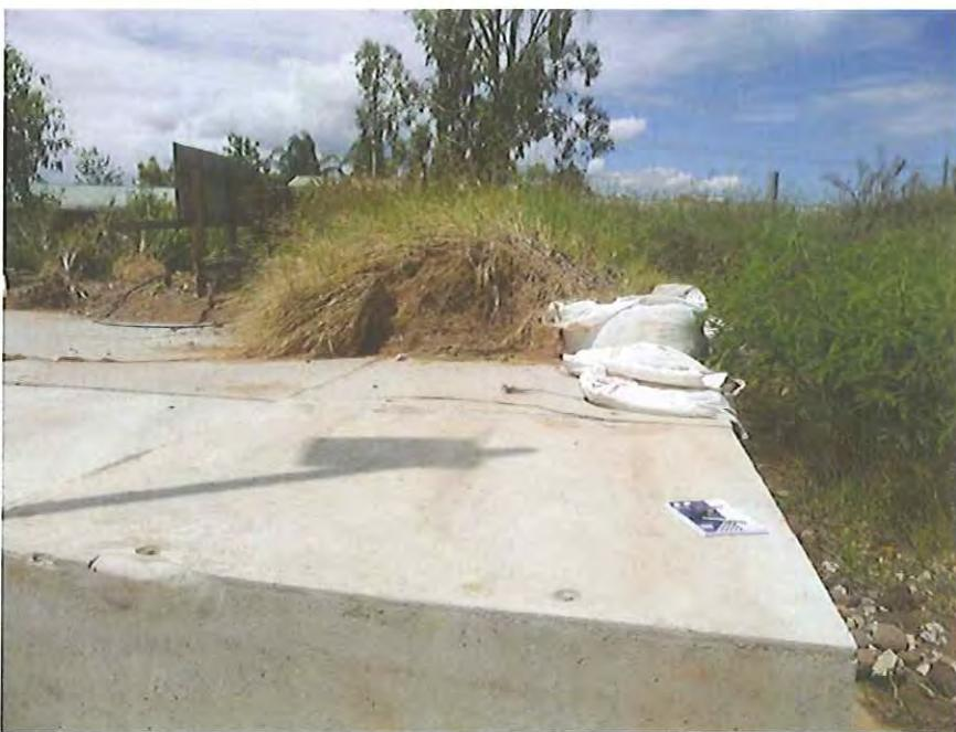
**Photograph A2** – Right abutment of damaged basin, showing remains of the embankment
