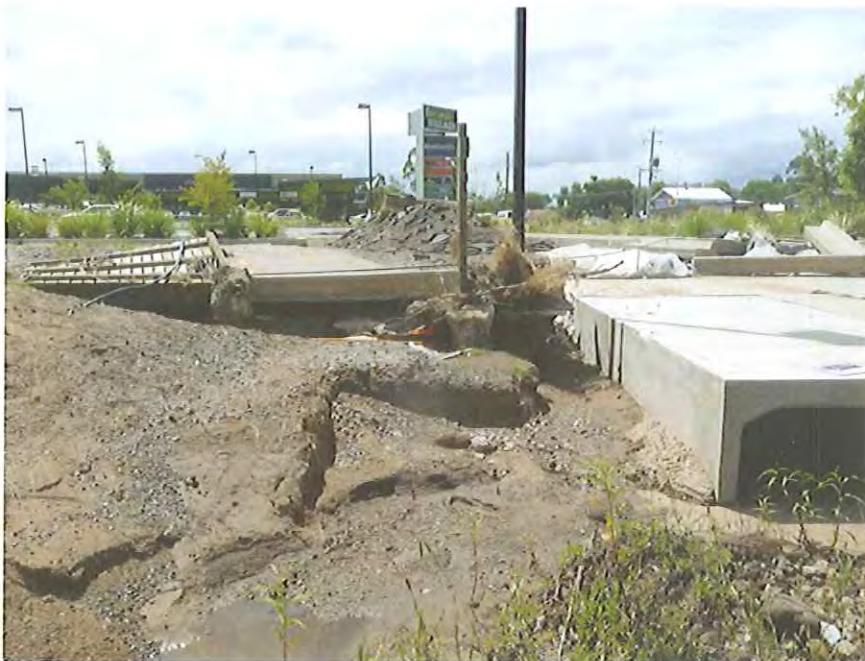
**Photograph A3** – Looking at the damaged left abutment of the detention basin, damaged car park pavement is evident in the background.
