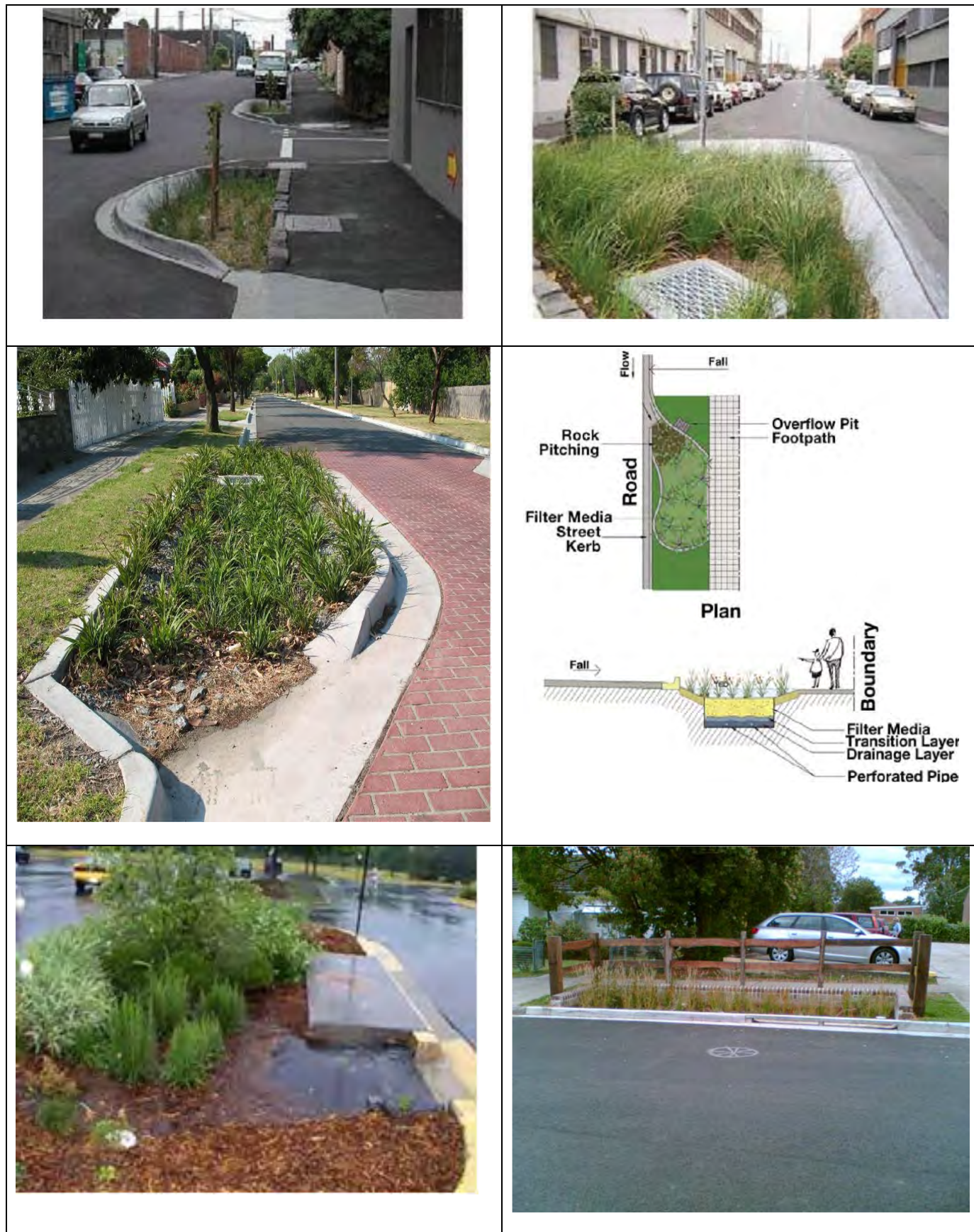
Figure 5.1 Examples of Roadside Bio-Retention Areas
