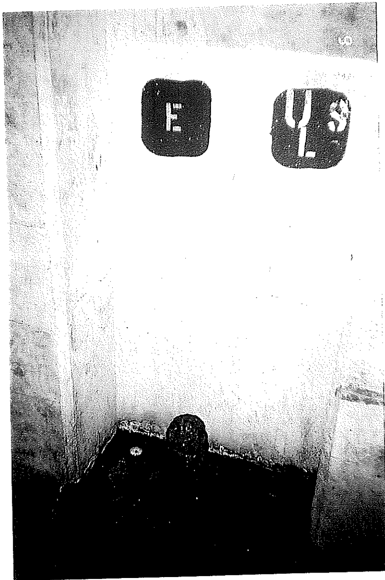
Contraction Joint Drain in Monolith S lower gallery - Note that in 1977 a horizontal crack was found in the upstream face of the dam at about RL 97.2.
