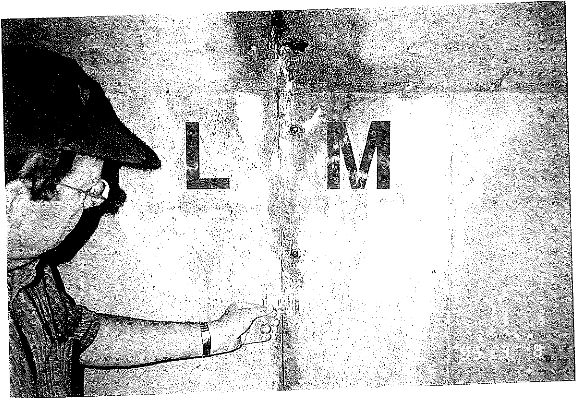
Seepage through Joint L/M - Water entering about 2 m above gallery floor.
