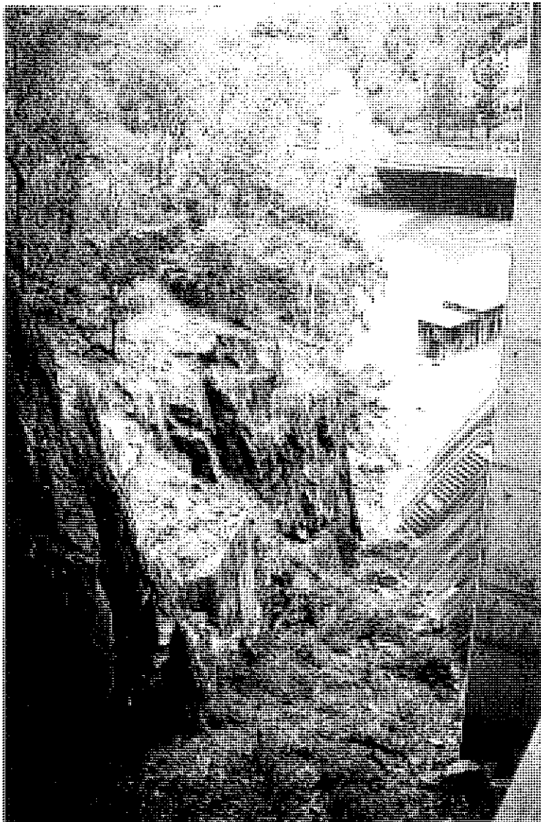
Right Abutment Stilling Basin Walls - Note weep holes, rock outcrops counterweight slides for spillway gates, signs of weathering "alkali; aggregate reactivity" in gate pier, backfilling behind retaining walls, stilling basin baffle, rip-rap downstream of stilling basin.
