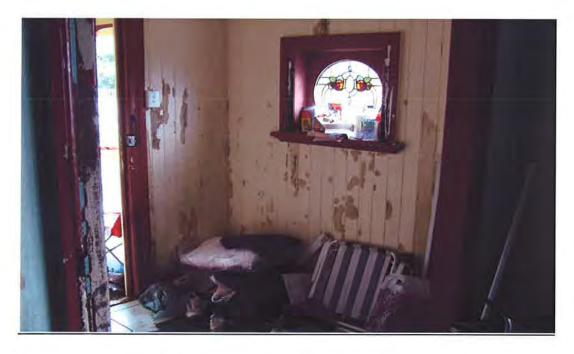
The internal wall that the stormwater has ran down.
