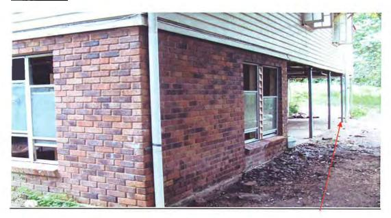
This photo shows the metal stump that the insured saw water coming out of.
