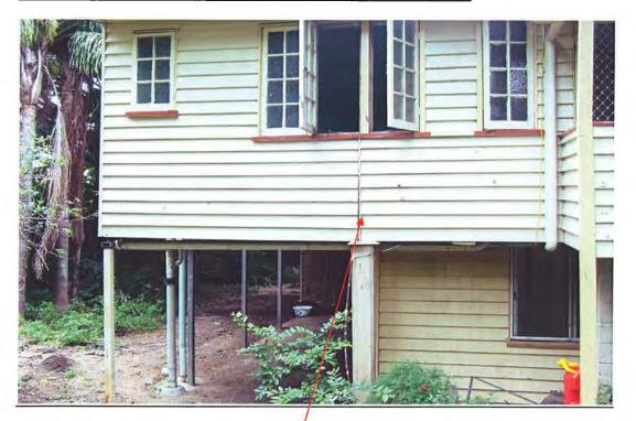
This photo shows the construction joint that the insured states has open up more due to the stump movement.
