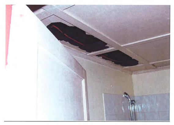
The bathroom asbestos ceiling that the volunteers have removed in the clean up.
