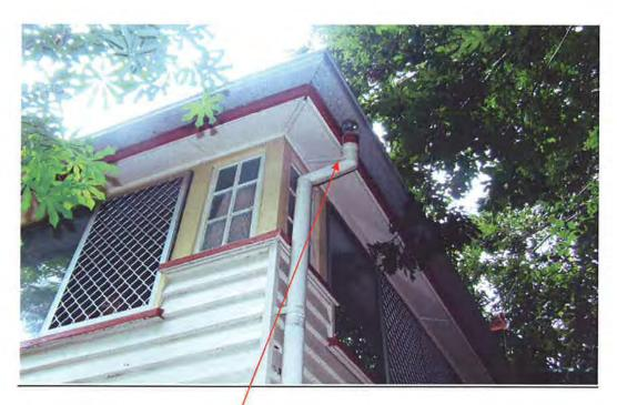
This photo shows the rear downpipe has dislodged from the gutter
