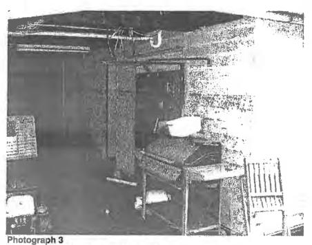
Outside area undemeath at rear of property - height of water on weatherboards
