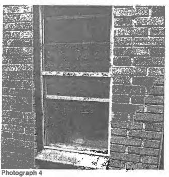
Rear downstairs bricked in area - shows height of water level.
