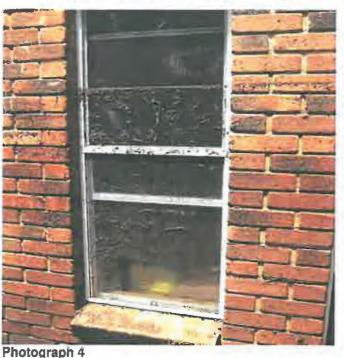
Photograph 4 Rear downstairs bricked in area - shows height of water level.
