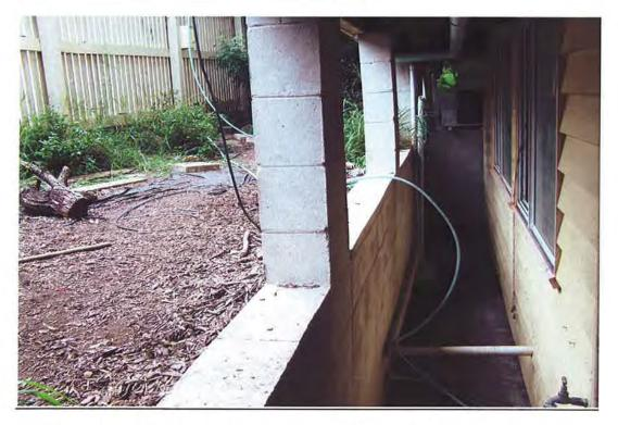
This photo shows the concrete block retaining wall/ stumps that are leaning.
