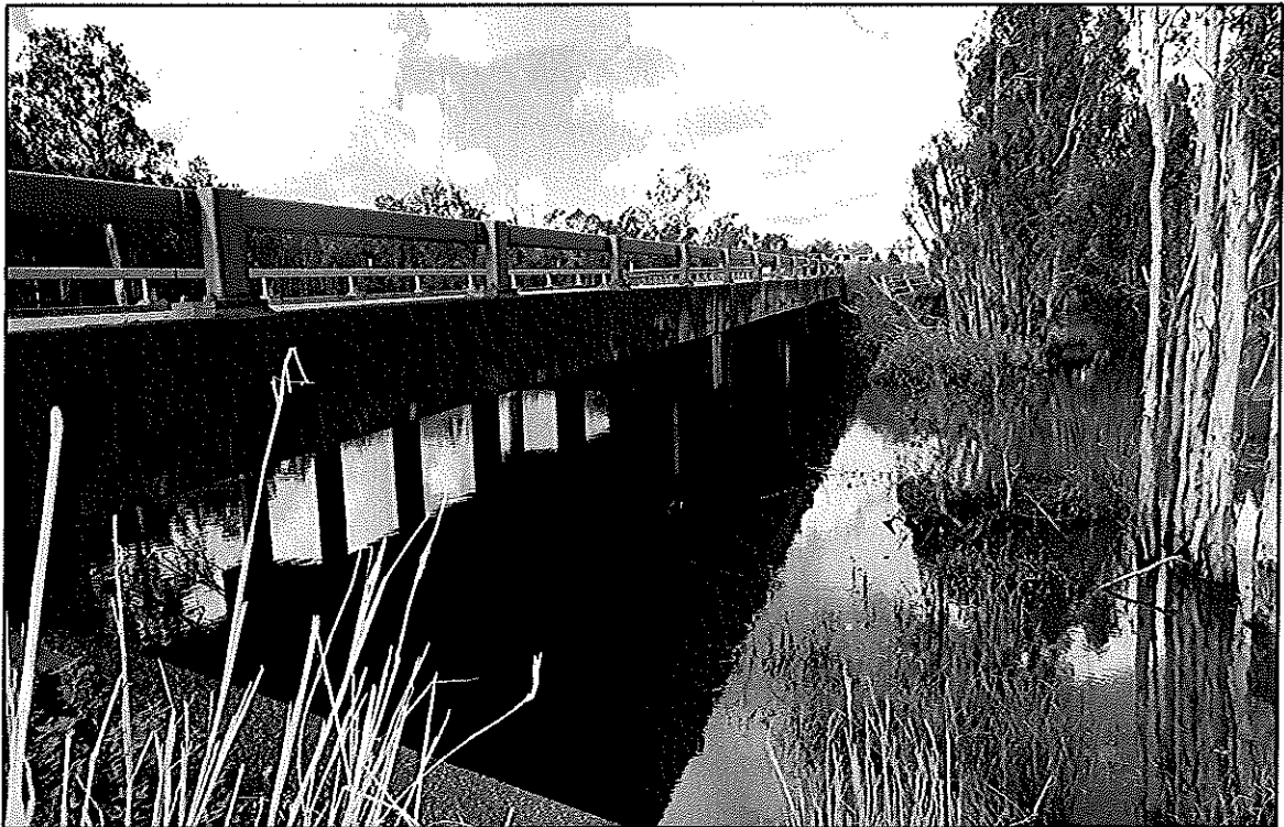
Figure 3.1 – Upstream Face of the Bruce Highway Bridge
