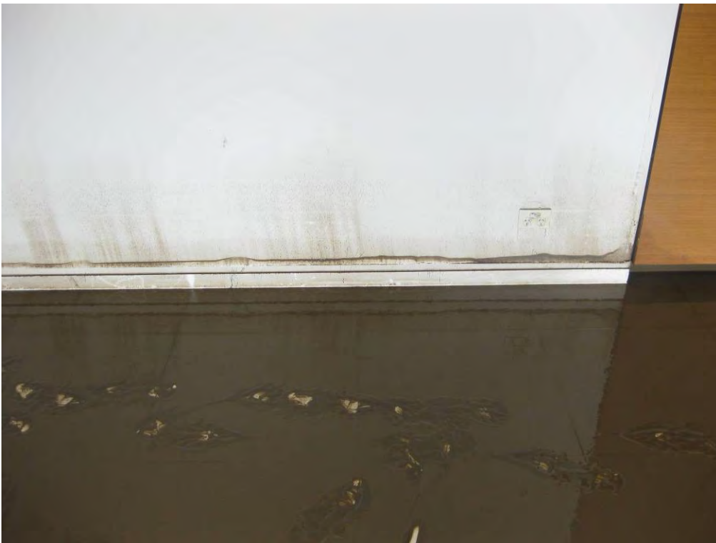
Figure: View of kitchen wall and pantry showing damage to plasterboard walls
