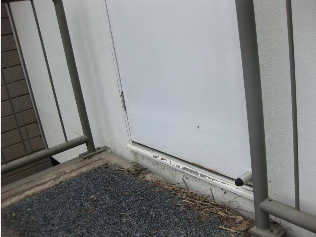
Figure: View from stairs on the eastern side of the sales office that shows the water line below the door
