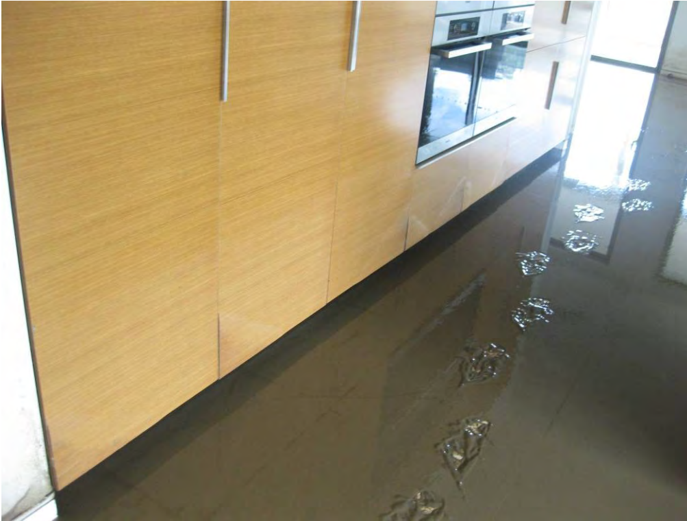
Figure: View of kitchen pantry showing warping of timber veneer
