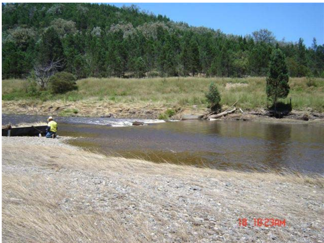
Gauging Station silted up and requires to be desilted to re-activate the gauging instruments
