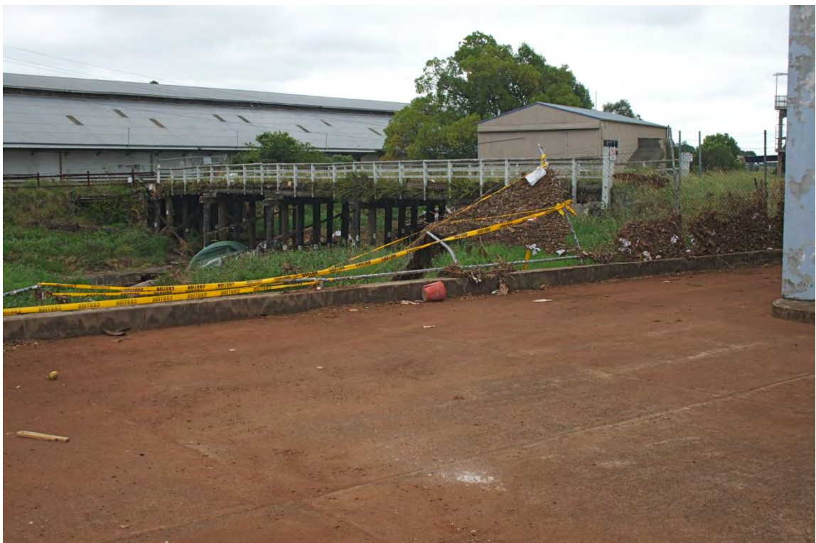
Photo No. 12 Gowrie Creek at Junction of East and West Creeks From East Creek Waterway Crossing: Floodwaters 2 m Above Deck Level
