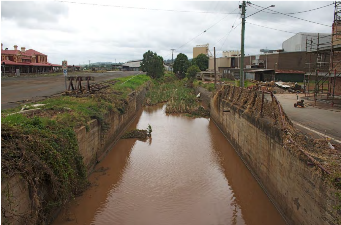
Photo No. 11 West Creek North of Russell St, Looking Downstream (Flour Mills in Background): Extensive Inundation Along Russel St.
