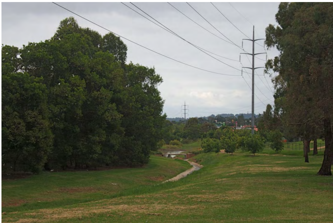
Photo No. 7 West Creek at Spring St Looking Downstream: Grassed Waterway with Concrete Low Flow Channel.
