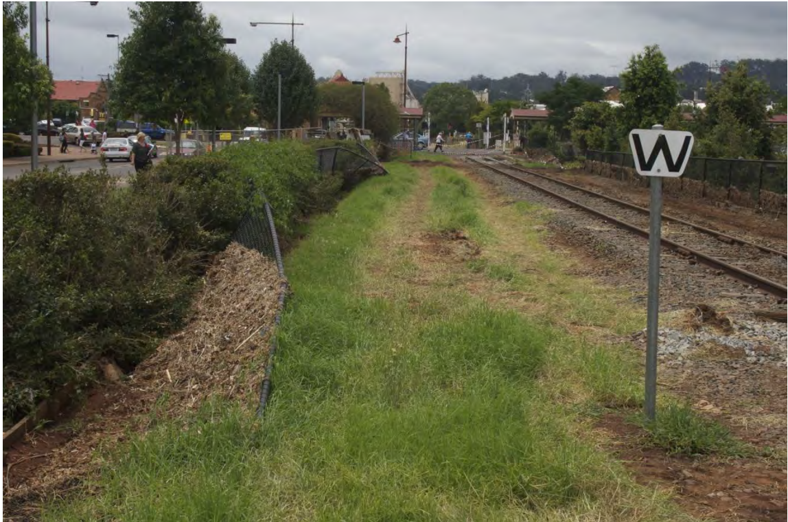
Photo No. 9 Looking North Along Railway Line Opposite Dent St (LHS), Russell St Crossing in Background: Northward Flowing Floodwaters from Dent St Flowed Eastwards across Railway Embankment and Back into West Creek (RHS Out of View)
