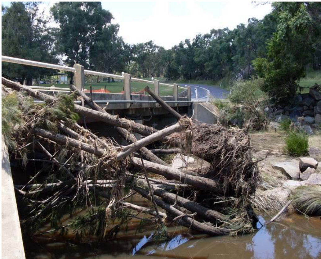
Down stream access bridge damaged and blocked with debris
