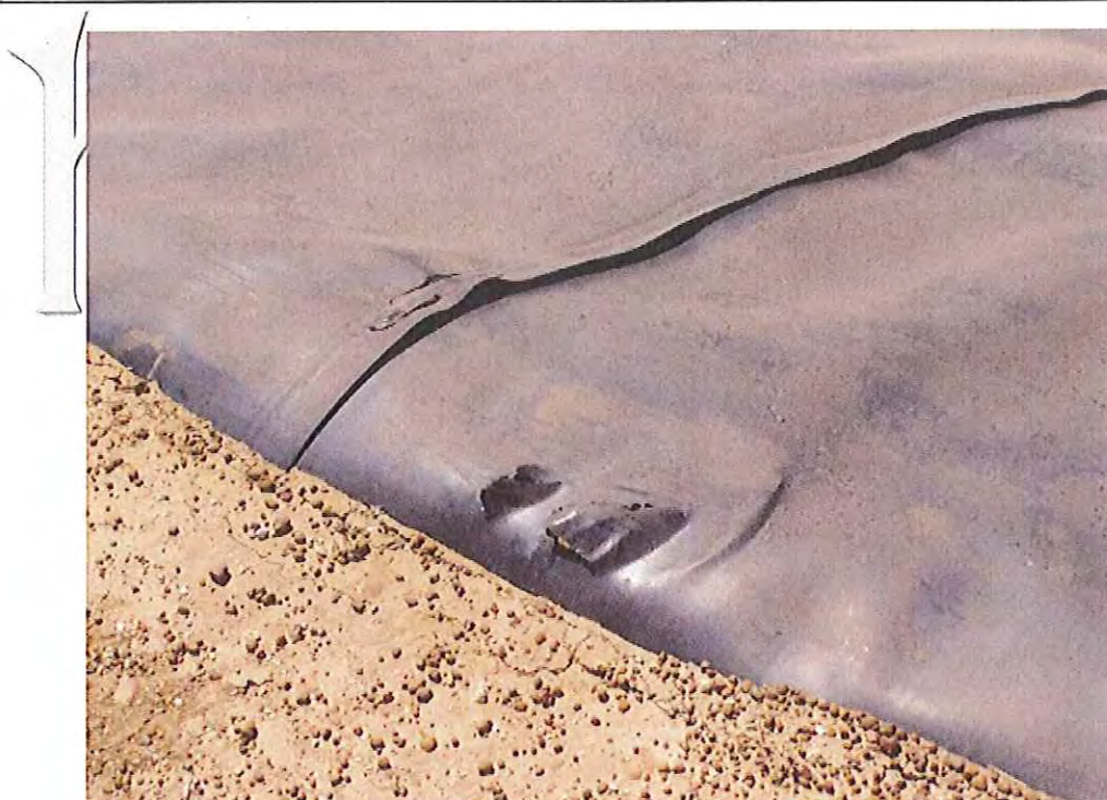
Photo 3-2: Dam1, tear in liner at northern crest
