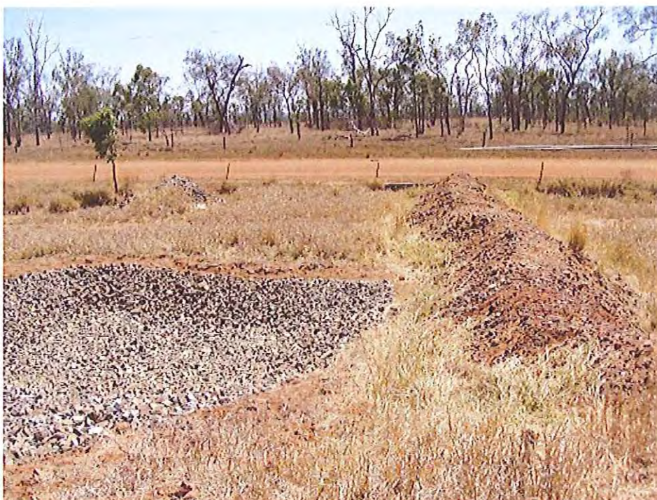
Photo 3-7: Dam 1, spillway stilling basin
