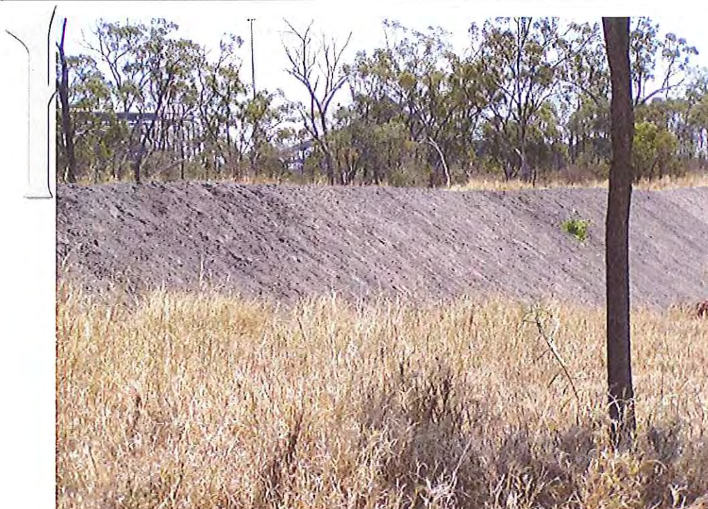
Photo 2-3: Environmental Dam, downstream batter
