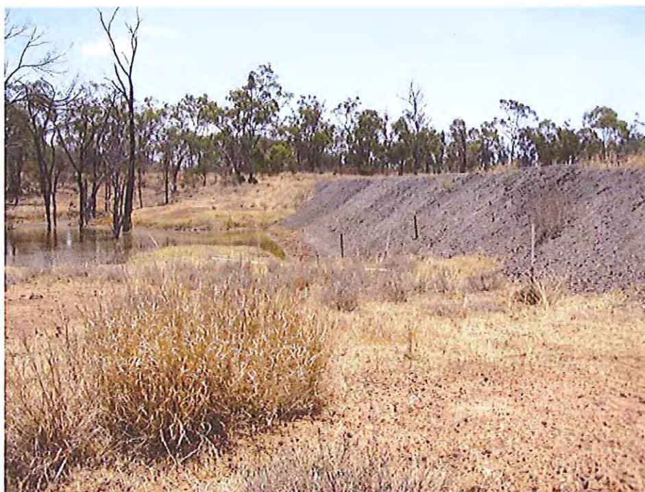
Photo 2-2: Environmental Dam, upstream batter
