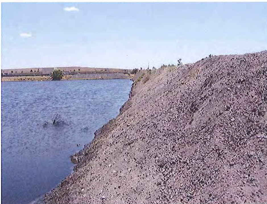
Photo 1-2: Production Dam, upstream batter
