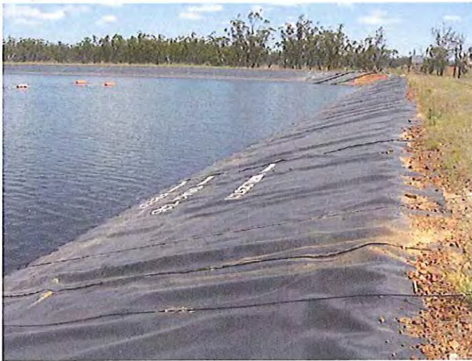
Moranbah North Dam 4 showing marked DSA and MRL level markings.
