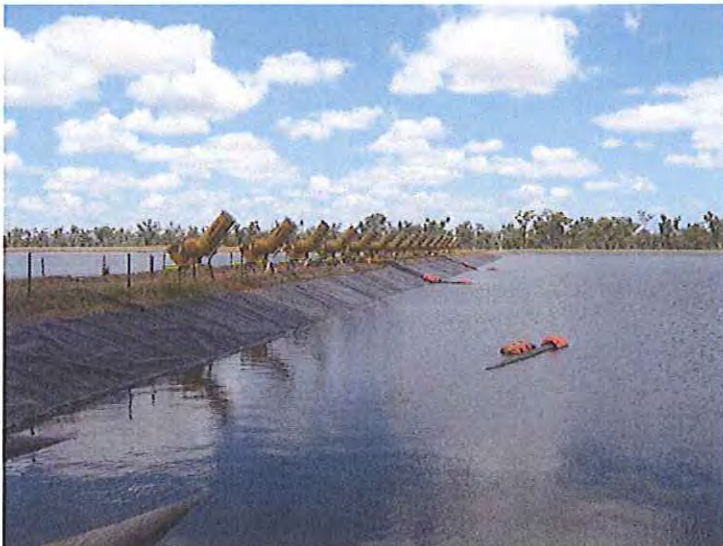
Moranbah North Coal Mine Dam 2 Liner in good condition.
