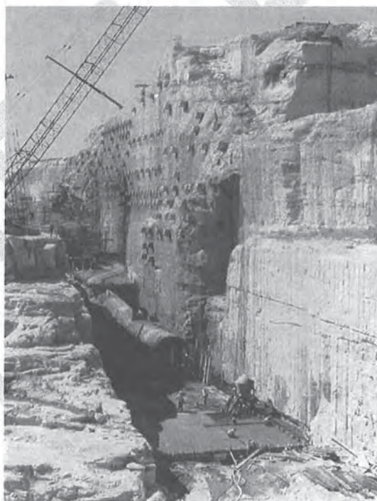
Photo 9- Wivenhoe Outlet and Spillway Plunge Pool Construction
