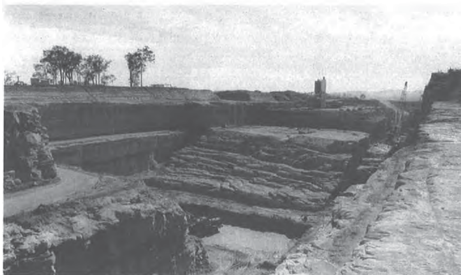
Photo 8- Wivenhoe Outlet and Spillway Plunge Pool Construction
