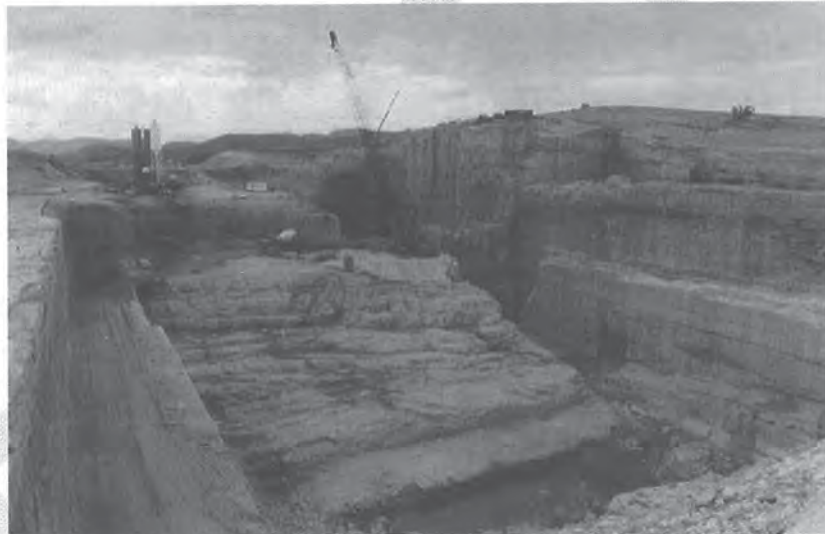
Photo 7- Wivenhoe Outlet and Spillway Plunge Pool Construction
