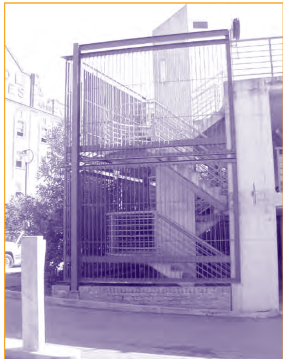
Figure e Casual surveillance of this stairwell is facilitated through location, design and selection of materials.
