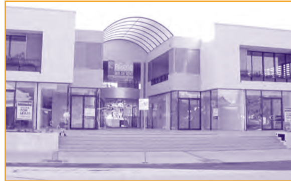
Figure g This building exterior provides excellent casual surveillance opportunity to and from the street, and also defines private from public space.
