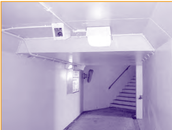
Figure s Risks associated with predictable routes such as underpasses can be alleviated with generous path width, use of surveillance technology, and the presentation of excellent levels of lighting, light coloured walls and signage
