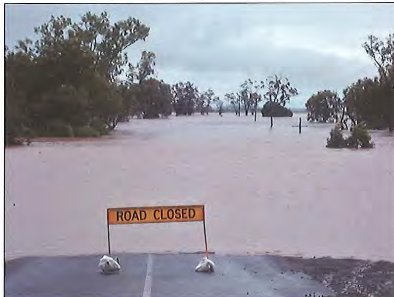
Plate XIX: Oakey Ck. at Jondaryan Woolshed midday 11.01.11 with water still rising. Under the water is the newly constructed Oakey Ck bridge designed to withstand a 1 in 100 year flood ! Power lines on right of bridge are just visible. Photo by G. Cooke.
