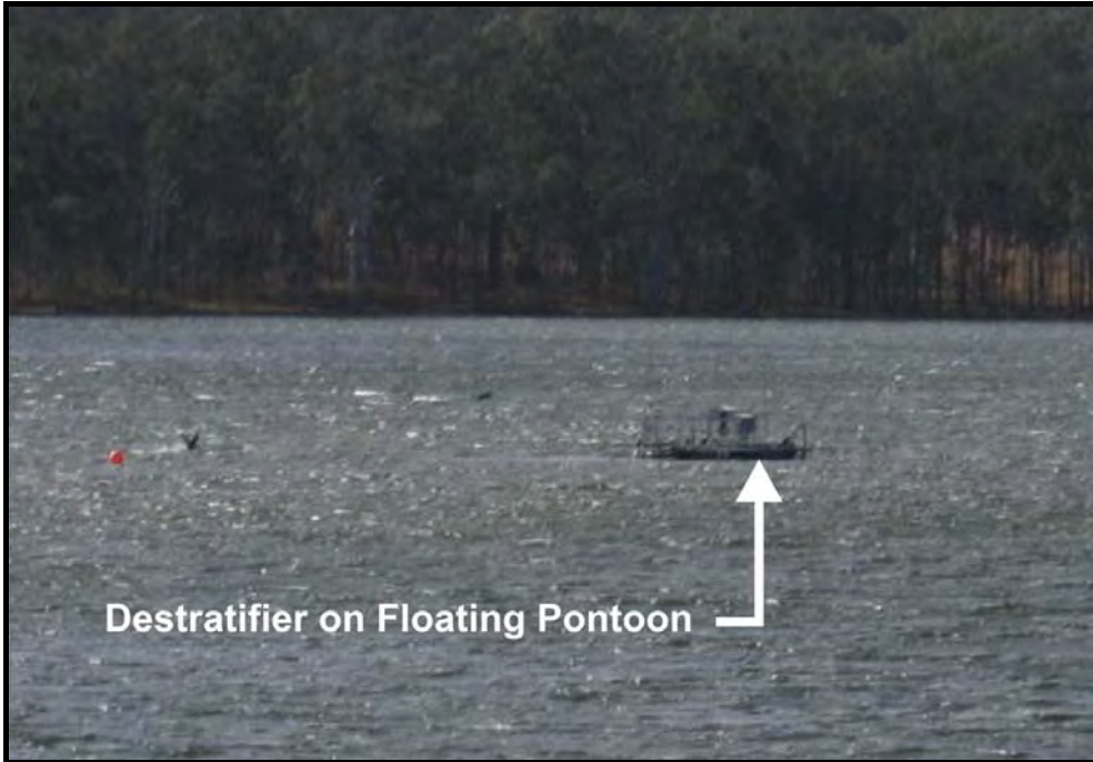
Figure 2-27 Destratifier (Picture taken from the Intake Tower)
