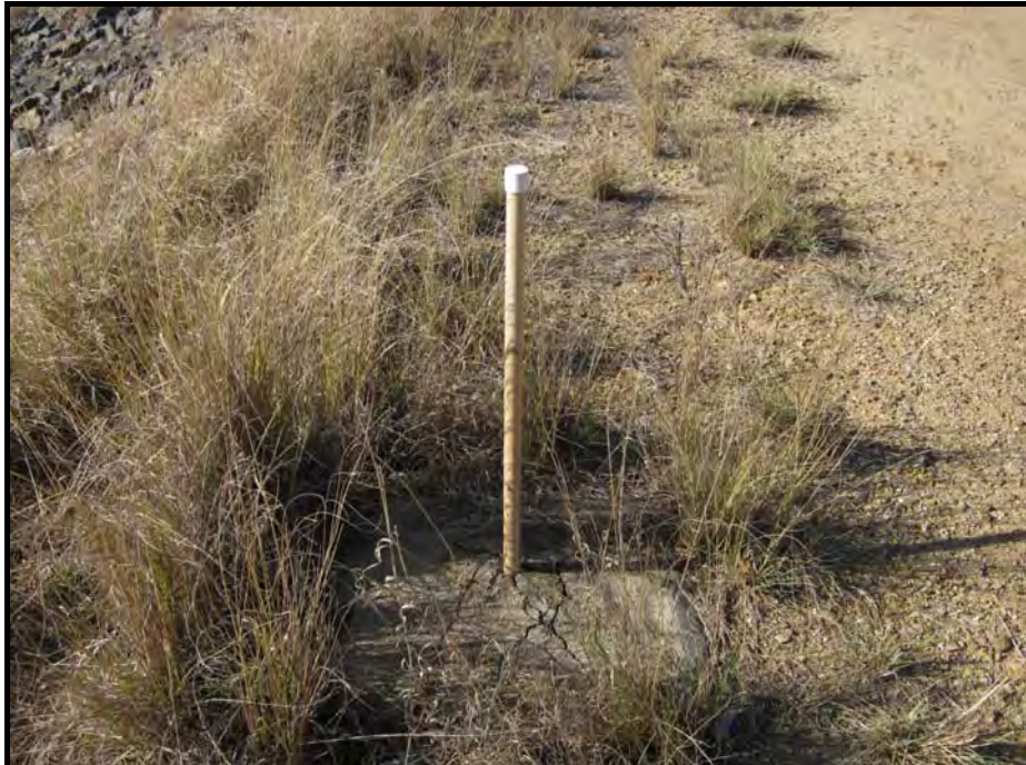
Figure 2-19 A typical standpipe
