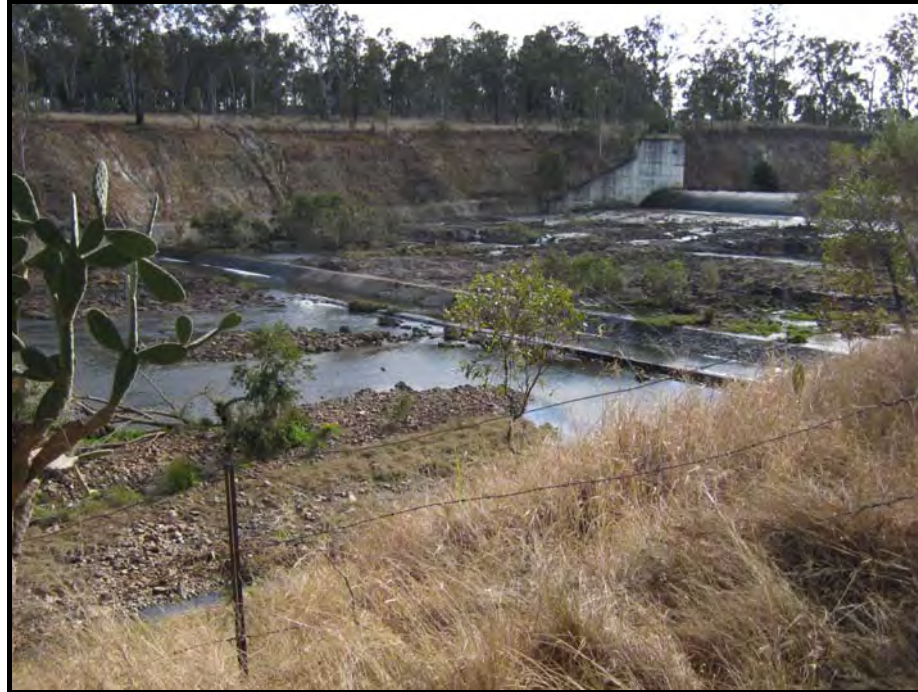
Figure 2-26 The Spillway Chute
