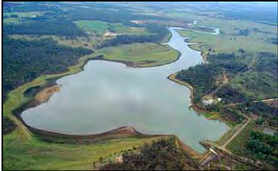
Figure 1-1 Aerial view of the dam.
