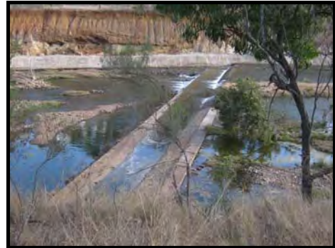
Figure 2-4 Drop Structures
