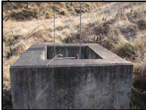
Figure 2-17 Diversion conduit outlet pit
