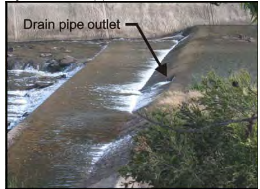
Figure 2-18 Drain pipe outlet i
