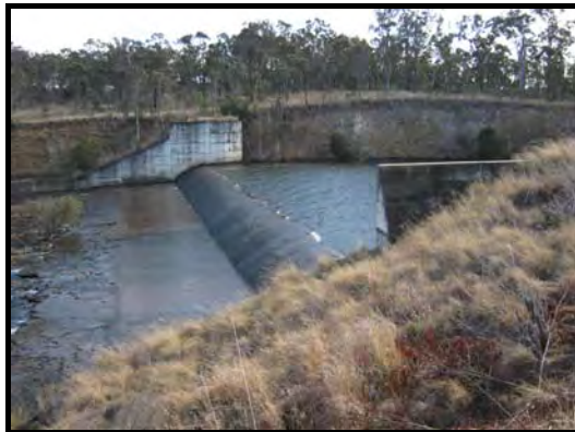
Figure 2-24 The spillway
