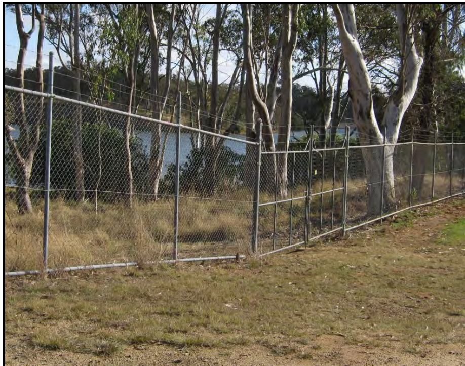
Figure 2-28 Security gate and fence
