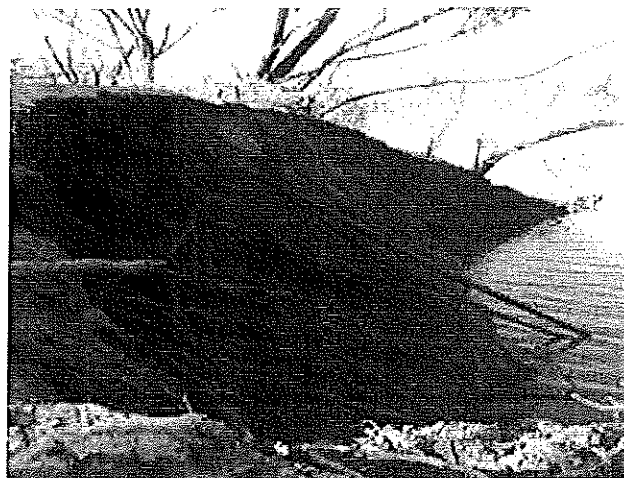
Photo 006 – Jan 11 Pump Site Riverbank Slump After
