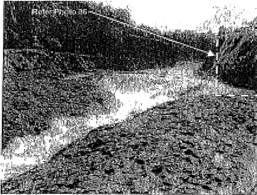
Photo 36 Undermining of left side spillway cut
