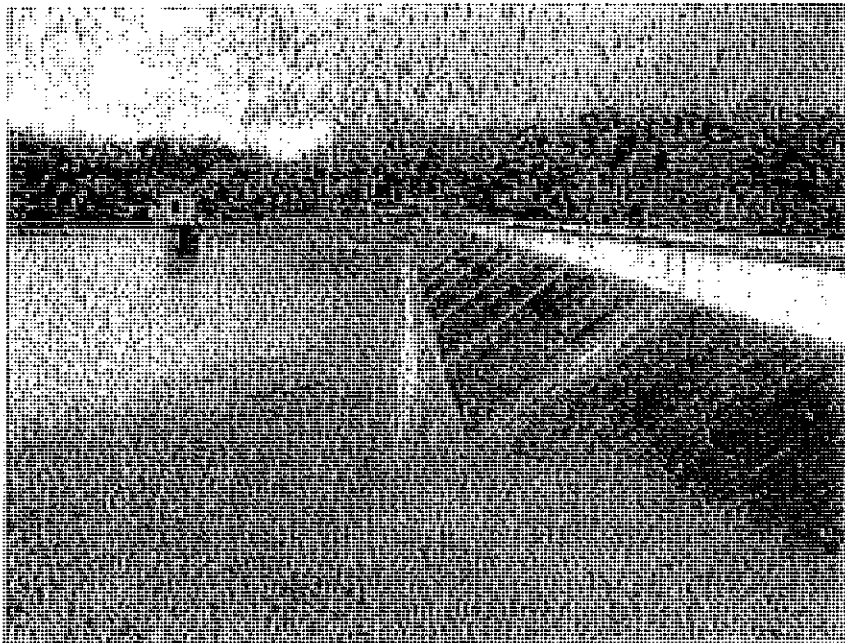
Photo 2 Upstream face of dam from right abutment (Note straight waterline)
