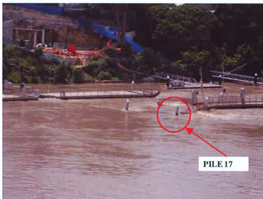
Figure 8 View of Mid section Pontoon under flood water
