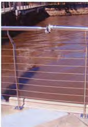
Figure 6 Handrail Spigot Failure
