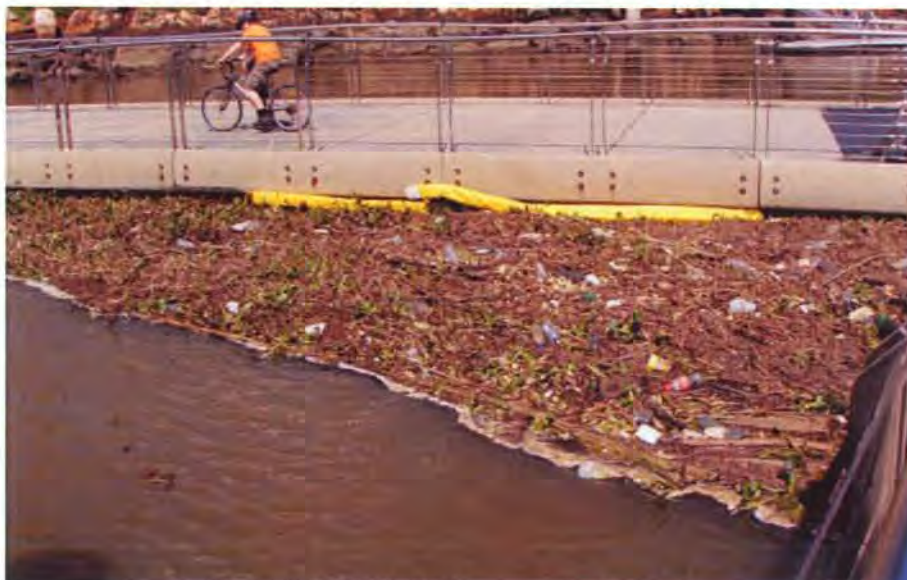
Figure 2 Debris Build up at Opening Section
