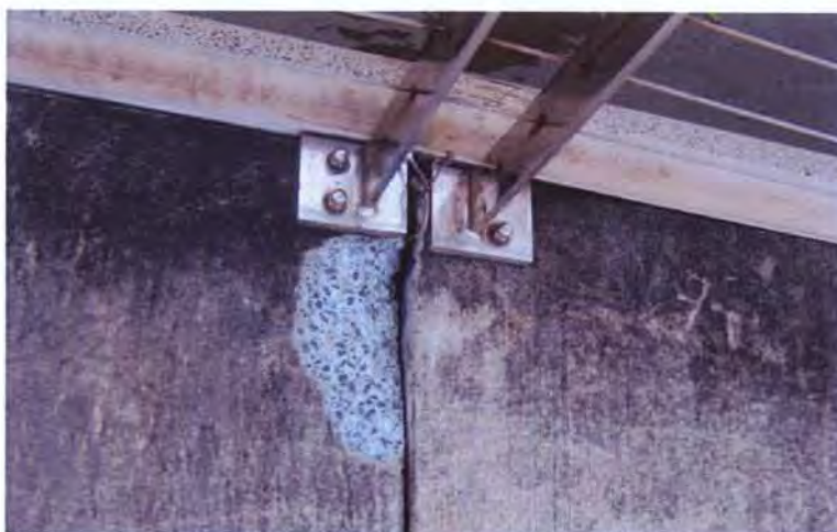
Figure 4 Concrete Spalling at Joints between Pontoons
